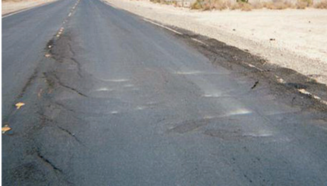
Figure 2.4 – Premature slippage failure on an overlay project in Nevada, USA (Charmot et al. , 2005)
