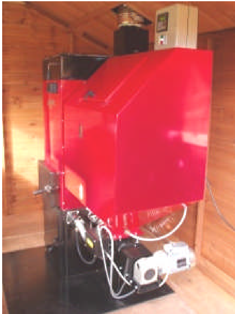
Figure 7.3: Photograph of Biomass boiler as installed for experiment
