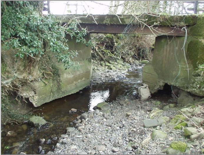
Figure 2.10 (a) Exposed bridge buttresses and (b and c) steep banks due to channel incision in the Upper Pontbren subcatchment.
