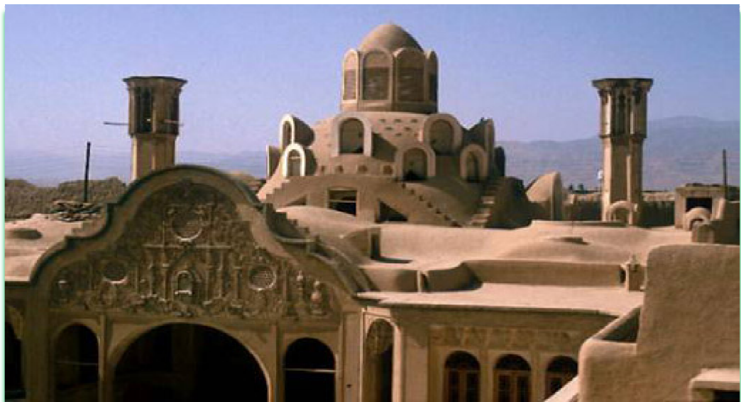
Figure 2.23 Borujerdi ha House wind catchers in Dolatabad Gardens, Yazd, Iran (Source ( http://commons.wikimedia.org/wiki/Category:Houses_of_Iran ))
