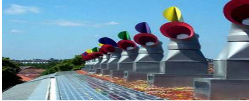
Figure 2.18 Photo showing a number of BedZED wind cowls in south London
