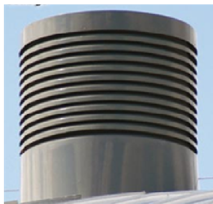
Figure 5.2 Modern design of wind tower (wind catcher)
