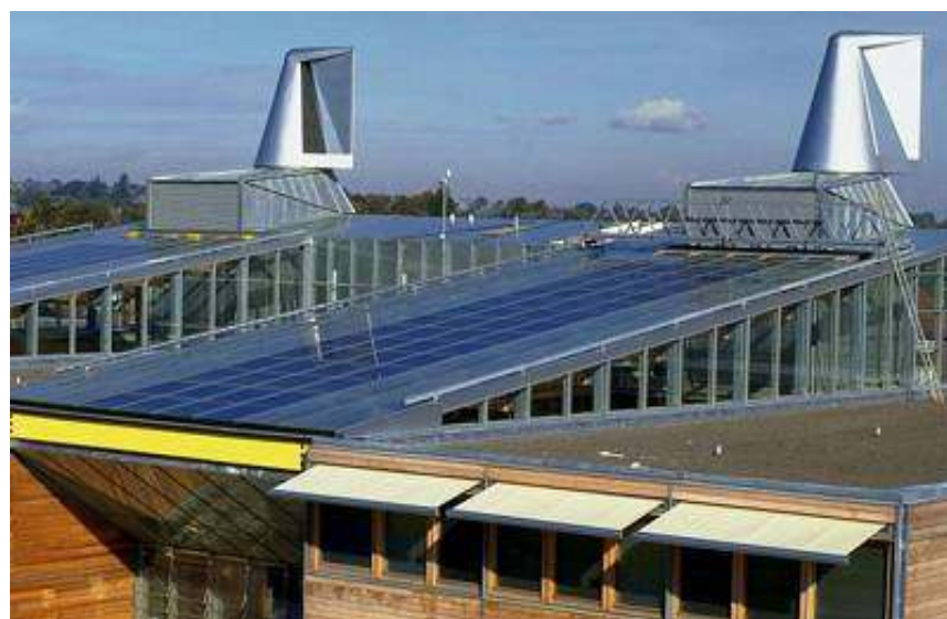
Figure 2.17 Photo of wind cowls at Jubilee Campus, University of Nottingham
