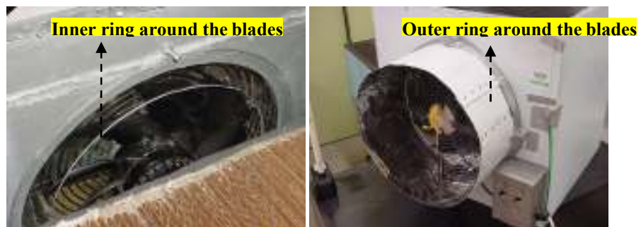
Figure 4.16 Photos showing adjustment to the fan inlet to prevent air leakage
