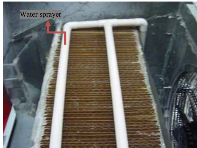
Figure 4.17 Water sprayer system using double tubing
