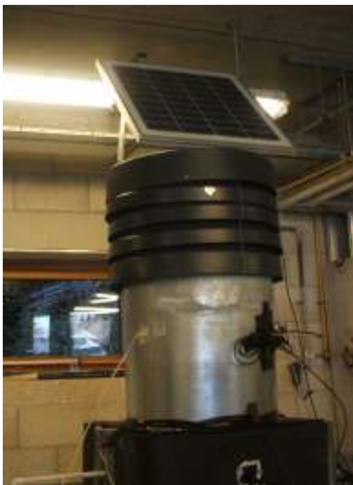
Figure 3.33 Operation of the system using solar power
