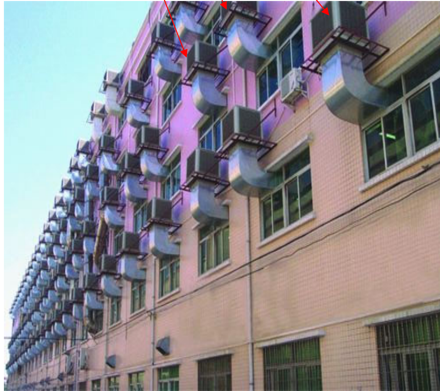
Figure 2.11 Multiple cooling pad evaporative coolers installed on a factory building
