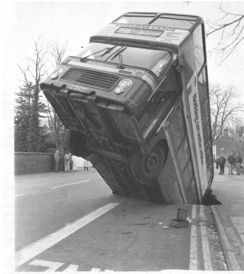
Figure 1.1 An example of (extreme) subsidence. Road collapsed beneath a bus, due to failure of weathered chalk above an abandoned mine, in Norwich, U.K. ( Waltham 1989 )
