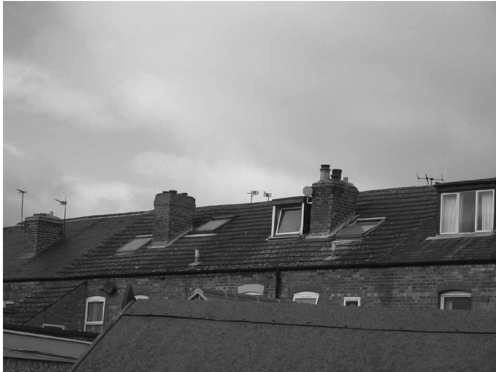
Figure 8-6: Variations in roof material and windows can make the effective emissivity difficult to determine with any certainty
