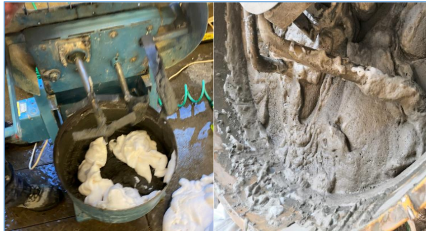
Figure 3.5: Foamed concrete production
