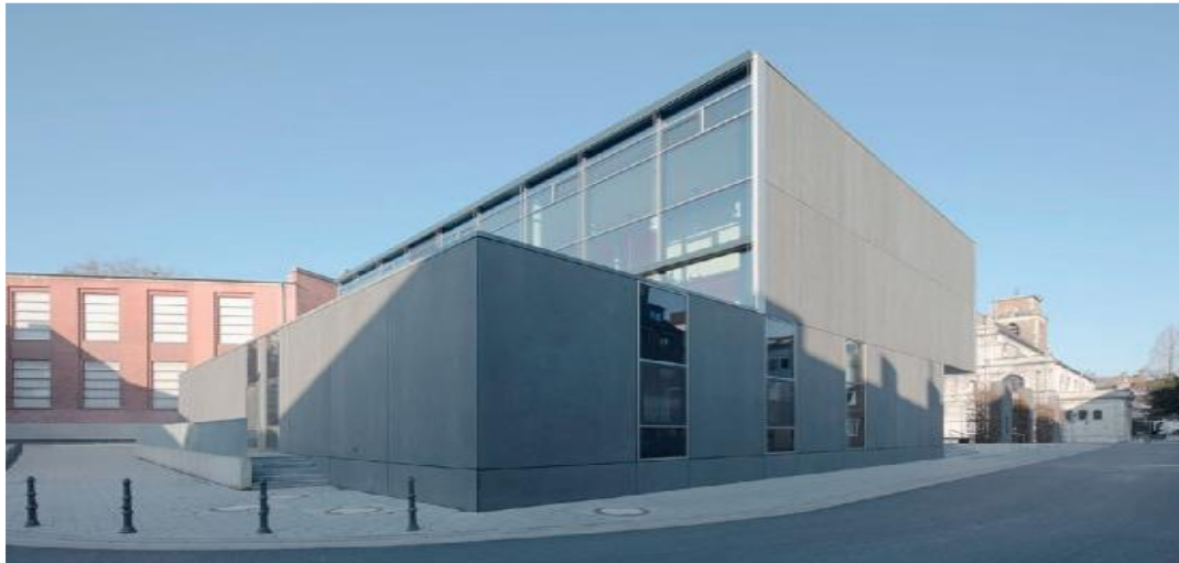
Figure 2.21: Large-sized TRC facade panels (Hegger & Will, 2016)
