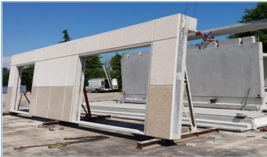
Figure 1.2: Multilayer cladding panel (Bamonte et al., 2017)
