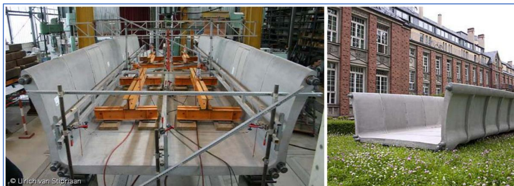
Figure 2.32: Textile reinforced concrete bridge (Curbach et al., 2006)
