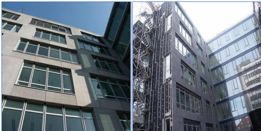
Figure 2.28: Office building, Dortmund, Germany (Curbach et al., 2006)
