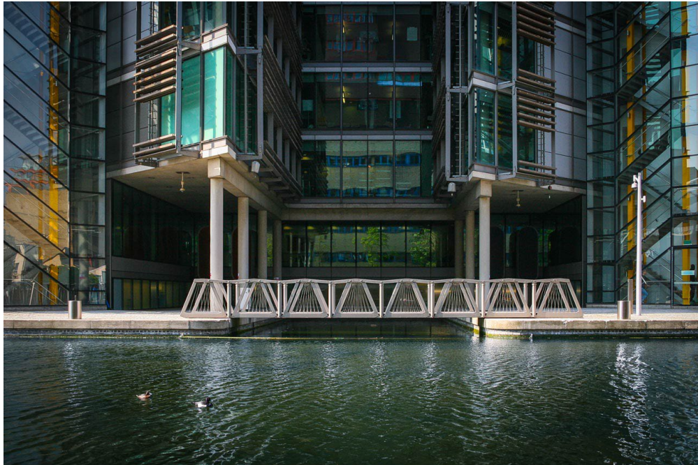
Figure 8.94: Heatherwick Bridge. Source: Littlehampton Welding Ltd.
