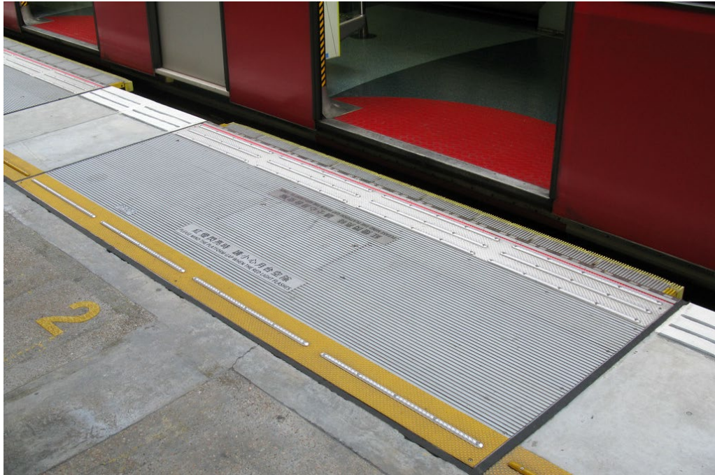
Figure 5.34: On-platform gap filler. Source: Wiki.
