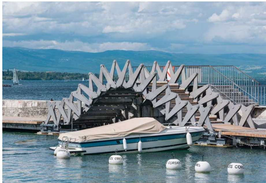
Figure 2.13: Jet d'Eau Bridge - raised state. Source: Ingeni.
