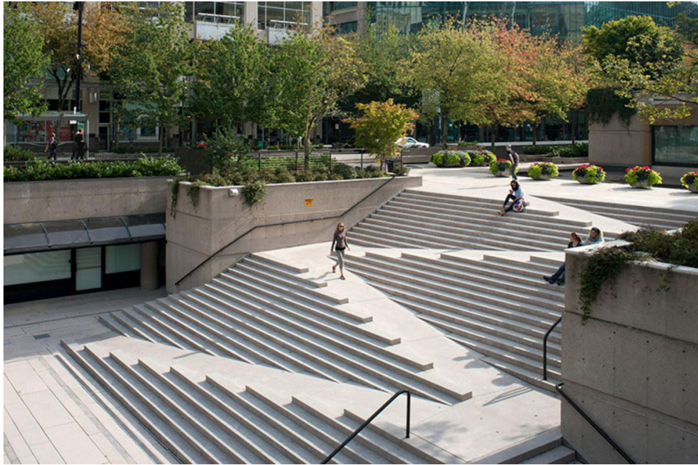
Figure 1.2: Ramps blended into public stairs in Vancouver. Source: Twitter.
