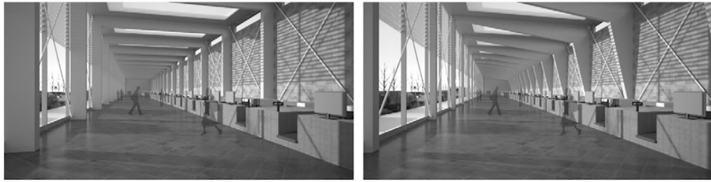
Figure 2.11: Two options for the design of the lateral and gravity structural system for an airport terminal: (left) a standard rigid frame and (right) a shaped rigid frame. The shaped frame uses a similar amount of material and creates a more architecturally expressive interior spaces.
