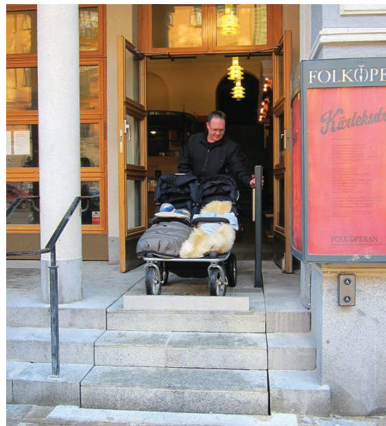
Figure 2.15: Stockholm Opera - the lifting platform in operation. Source: Guldman Co
