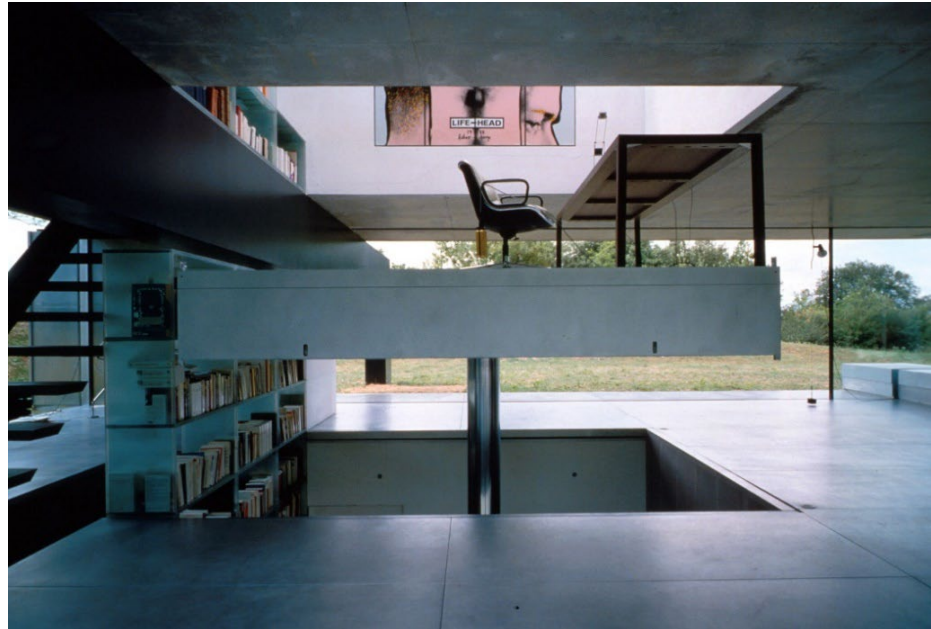
Figure 2.12: House in Bordeaux - a mobile platform allowing vertical navigation of wheelchair users in operation. Source: OMA.
