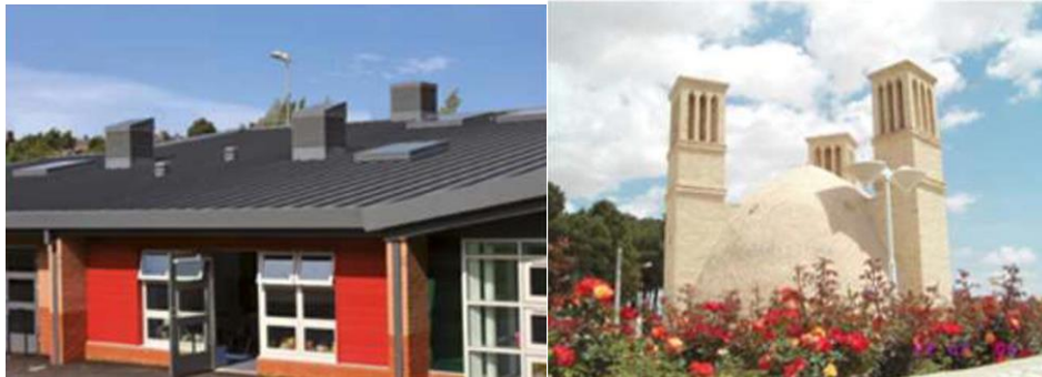
Figure 2.1 Photo of roof top windcatcher applications (a) in the UK [47] and (b) in Iran [48]
