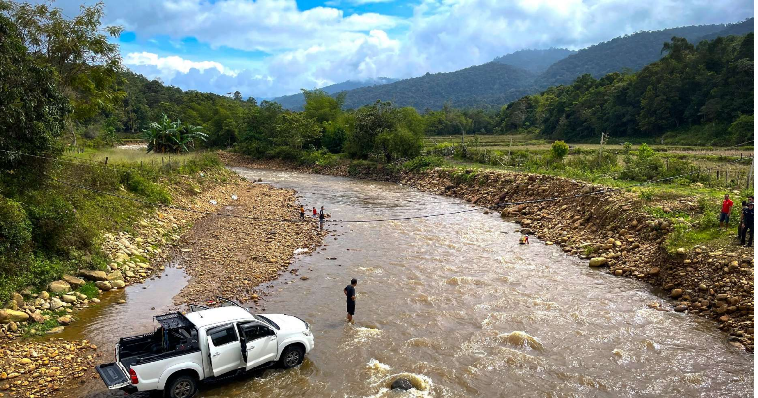
photo taken at Long Telingan showing channel re-alignment undertaken by the local following a large flood Photo: Yih Yoong Lip, February 2023
