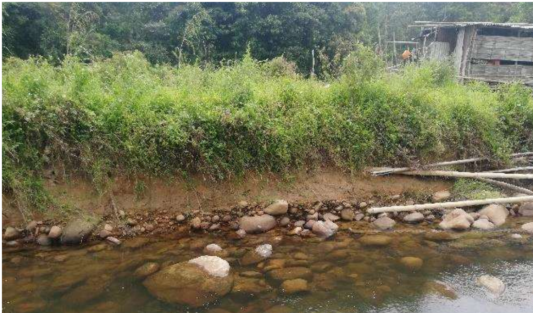
Plate 4.5: Bank after brush wall was washed away in December 2019 at Site A.
