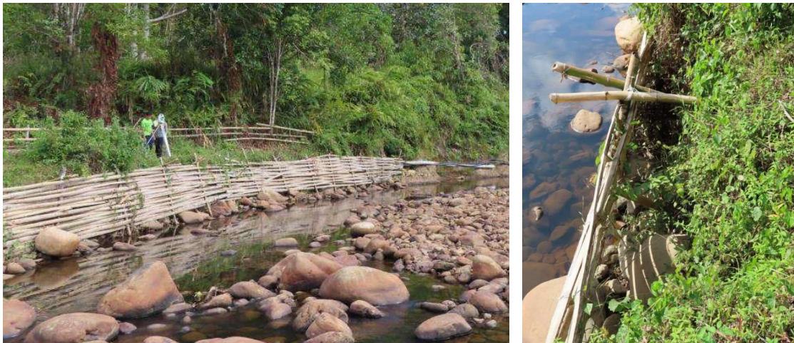
Plate 4.9: Live fencing at Site B. Left: completed installation of the bamboo wall with an extent of 40 meters. Right: close view of bamboo wall showing split bamboo (28 th September 2019, source from Belinda Lip).
