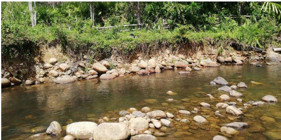
Plate 4.10: Eroded bank after the brush wall was washed away in December 2019 at Site B.
