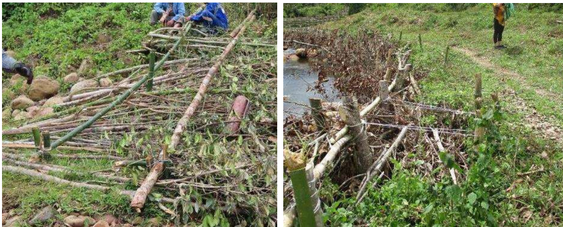
Plate 4.1: Brush mattress installed at the true left bank of Site C (left) and brush wall installed at Site A (right).
