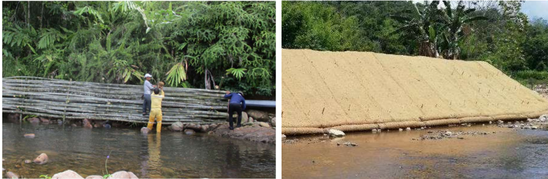
Plate 4.2: Bamboo fencing at Site B (left), Coconut geotextile mat installed at true right bank of Site C (right).
