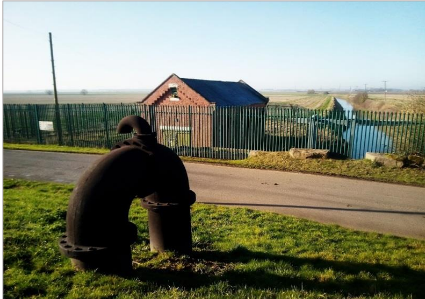
Figure 45: South Field Pumping Station on South Field Drain © Kathryn Bullen
