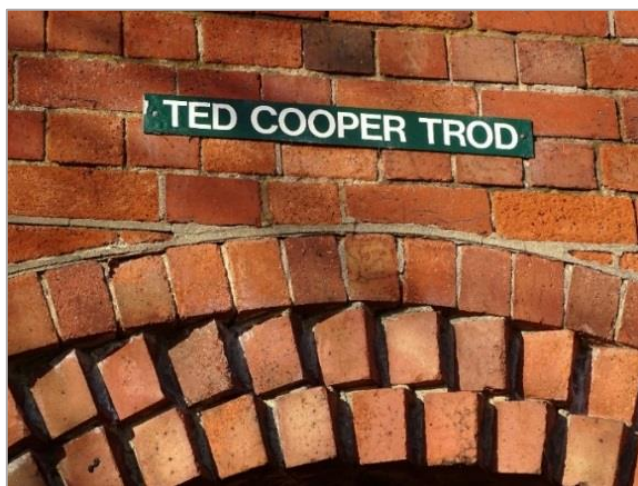
Figure 37: Ted Cooper Trod sign located on a path running under the disused Axholme Joint Railway in Haxey © Kathryn Bullen
