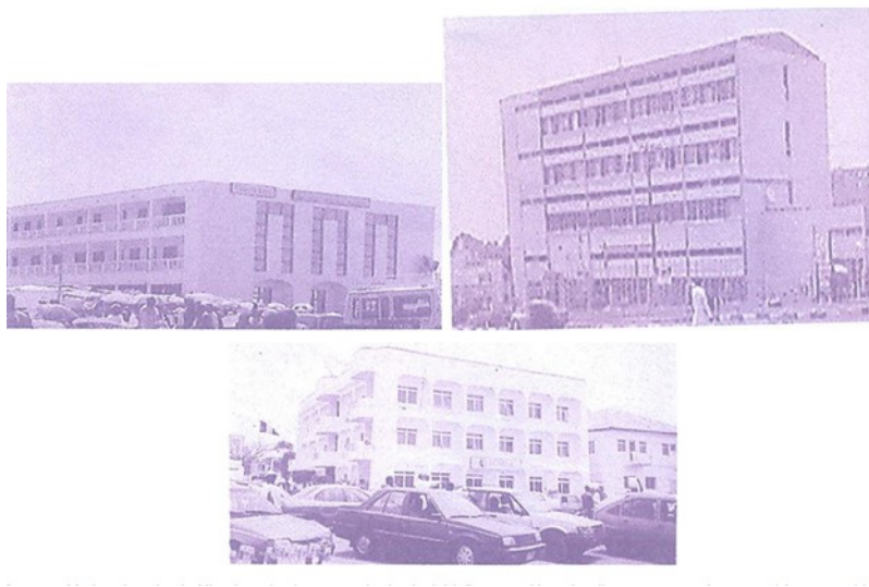
Figure 2-13: Modern housing in Nigeria arrived as a result of colonial influences. Note the disappearance of courtyard feature which is indigenous to Nigeria (Rikko & Gwatau, 2011: 276)
