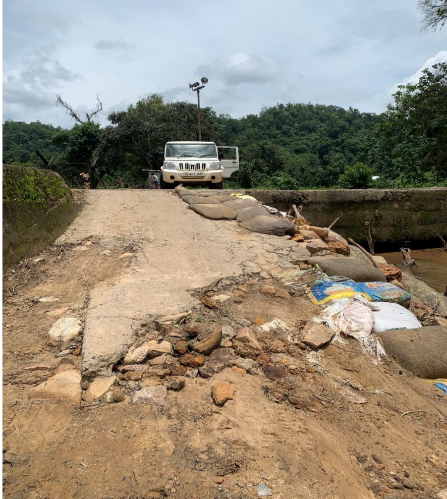
Figure 5.9: The remains of a road that leads to a stream that was washed away by a flash flood in August 2020
