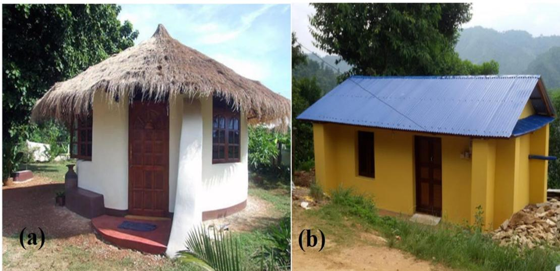
Figure 2-9 (a) thatched roofs and (b) pitched roofs on earthbag buildings [101]
