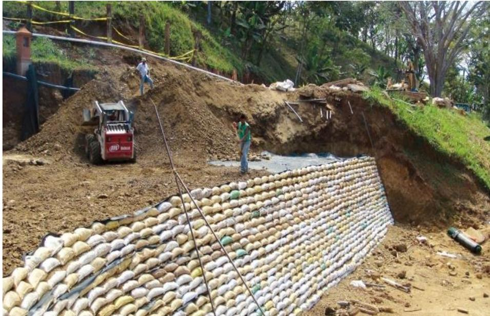
**Figure 2-4** Green retaining wall made with earthbags [81]
