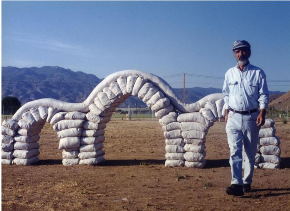
**Figure 2-5** Architect Nader Khalili during earthbag building demonstration [82]
