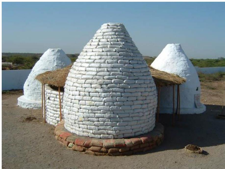
**Figure 2-8** Earthbag house with dome roof [99]
