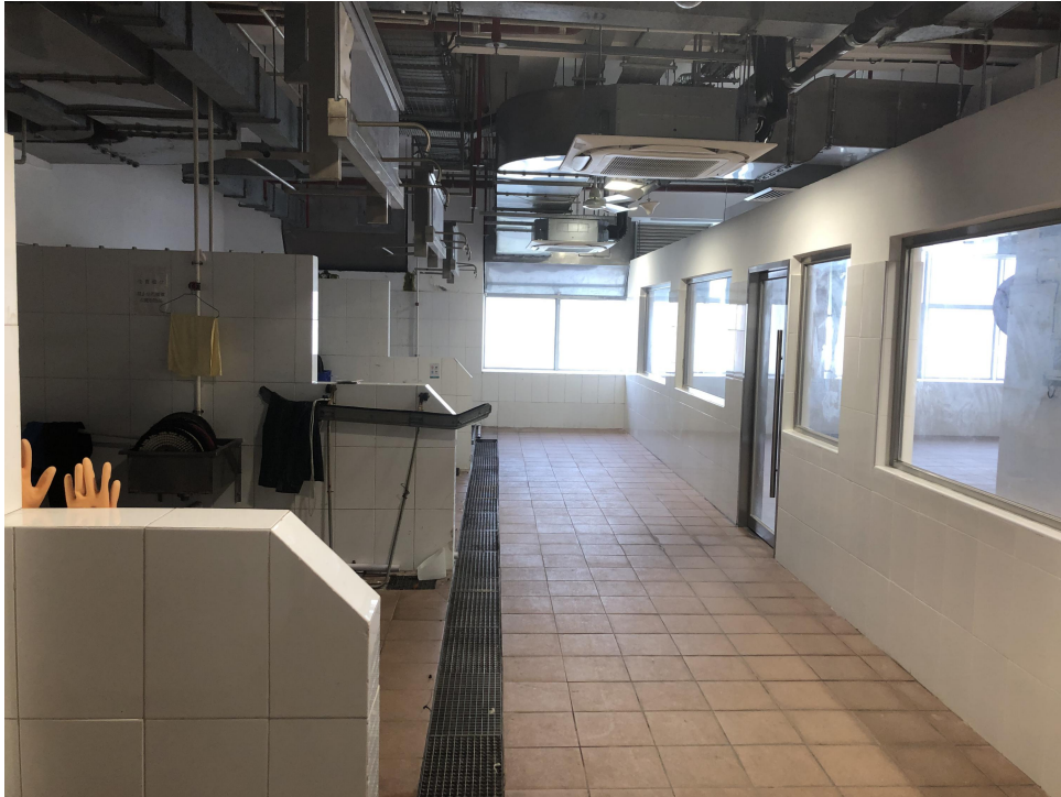
Figure 24. The current situation of the second floor of Shalitou market
