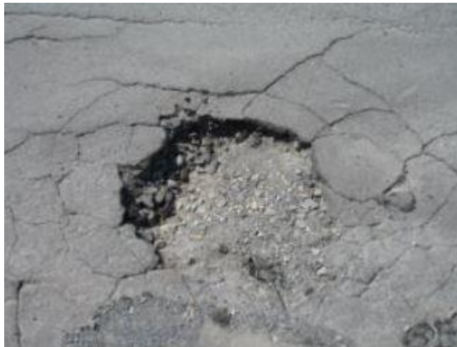
Figure 2. Fully formed pothole (Koch and Brilakis, 2011)
