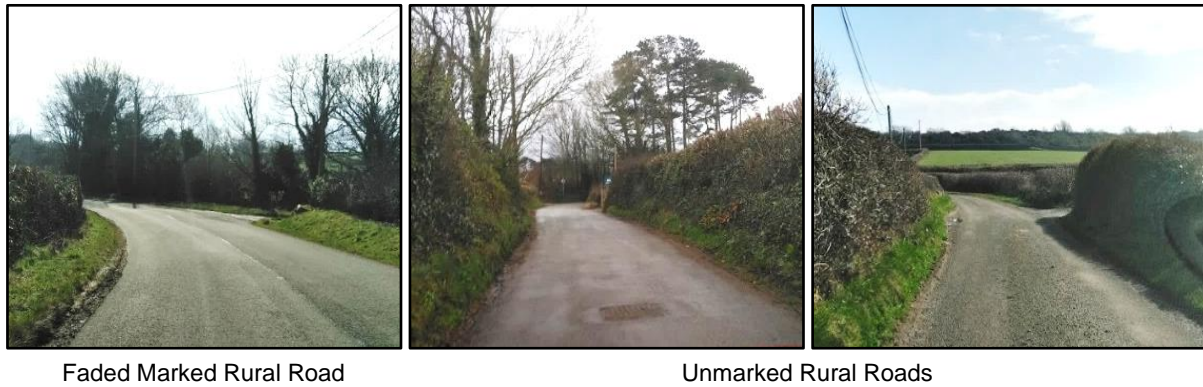
Figure 3.10 Unreadable rural roads (example photographs)
