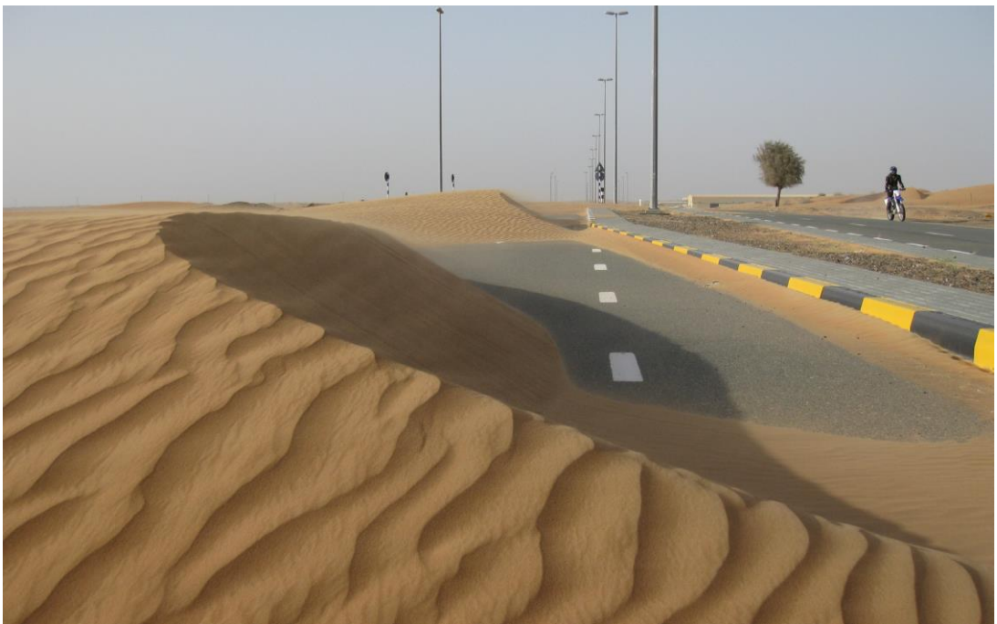
Figure 1.6. Migration of dunes across a newly constructed road (Photo credit: David Thomas).
