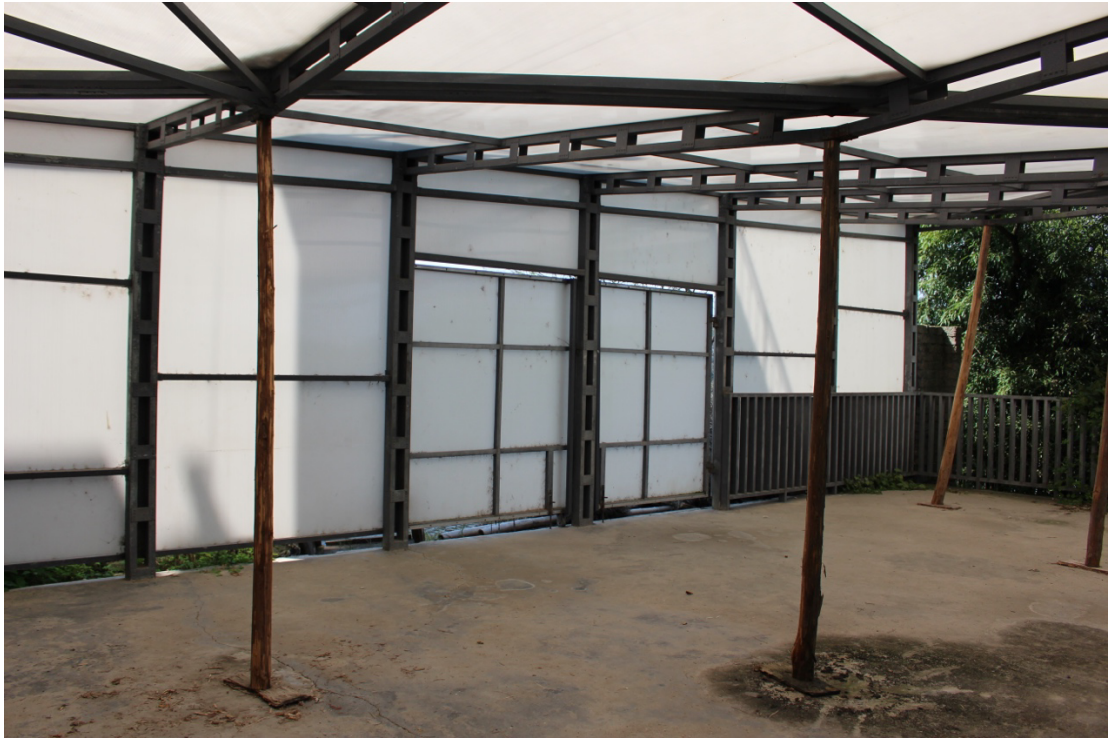
Figure 39. The classroom height problems caused by the increasingly structural subsidence; Wooden pillars are temporarily used for support (Photographs by author)
