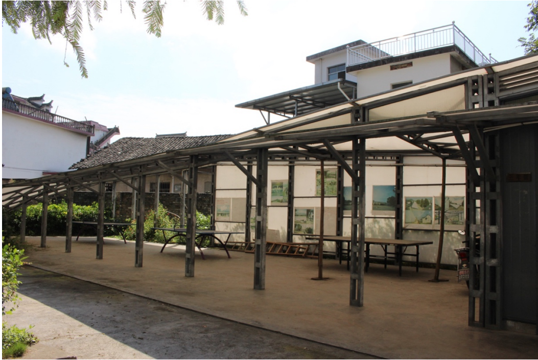
Figure 36. The activity room of the Xiuning Shuanglong Primary School with open light steel structures (Photographs by author)
