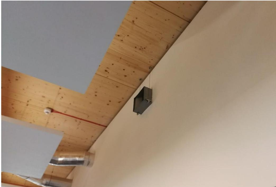
Figure 5-4 image of the air tunnel that extract the air from the small offices to the main open space office
