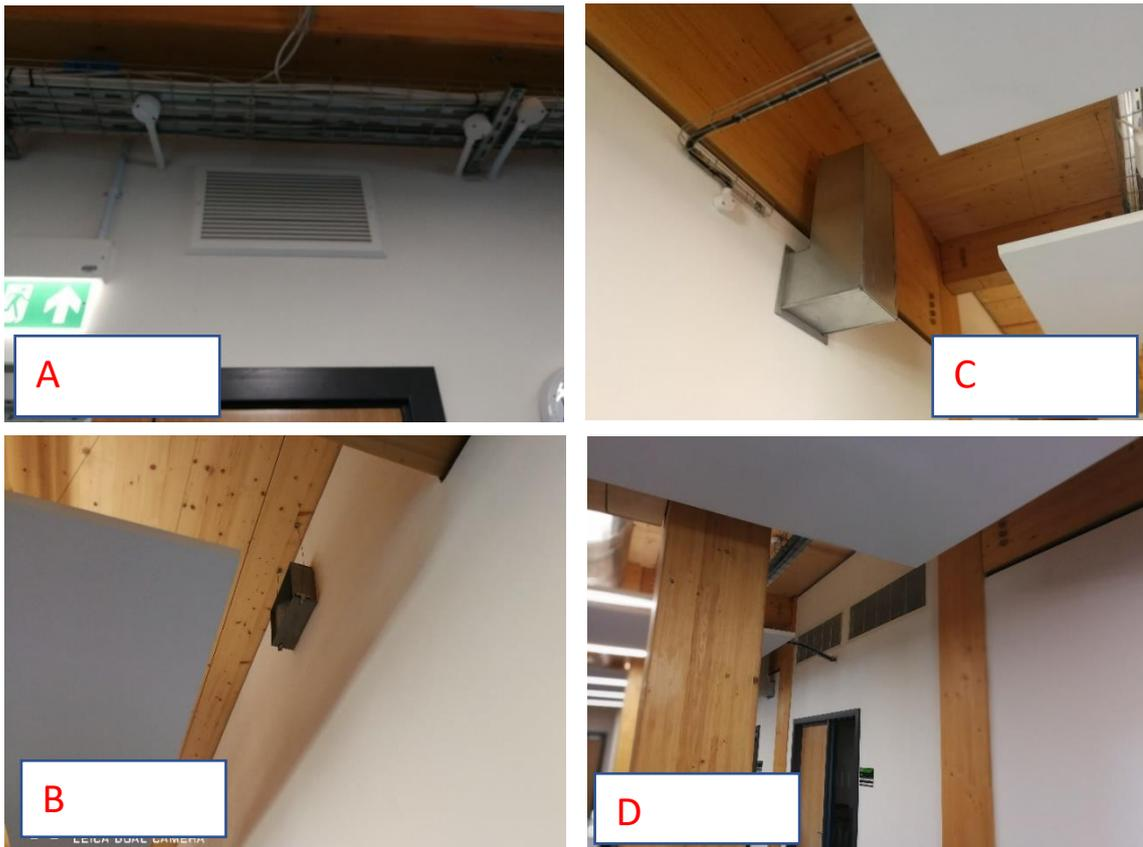
Figure 3-9 the ventilation system in the GSK chemistry building: A) the outlet grill, B) an opening that brings mixed air from adjacent offices, C) outlet of adjacent offices, D) extract grill
