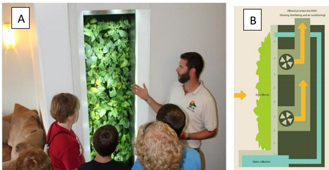
Figure 2-26 A. Novel biofilter unit installed in home for pilot study; B. An example of an original biofilter design for indoor applications [4-185].
