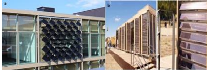
Figure 2.2. Different PV shading devices, (a) with a more aesthetical approach [91] and (b) with louvers design [92].
