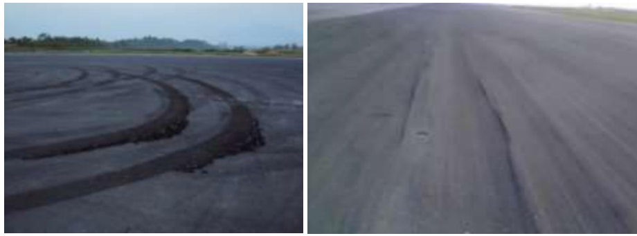
Figure 2.19 Premature damage and rutting after trafficking newly laid asphalt (Nepal 2014)
