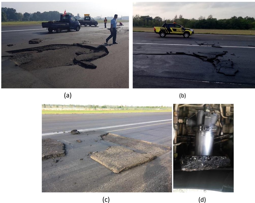
Figure 2.29 Slippage failure in new asphalt overlay layer at the runway in Indonesian airport: (a) Jakarta (HLP) airport, (b) Yogyakarta (JOG) airport, (c) Lampung (TKG) airport, (d) FOD found in aircraft body in Surabaya (SUB) airport (Courtesy of Indonesia Airport Authority).
