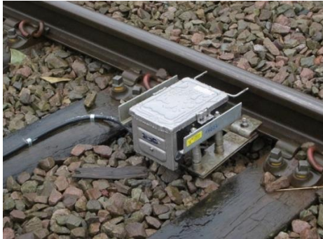
Figure 4-6 Directional Treadle used in AHBC Track Circuits.
