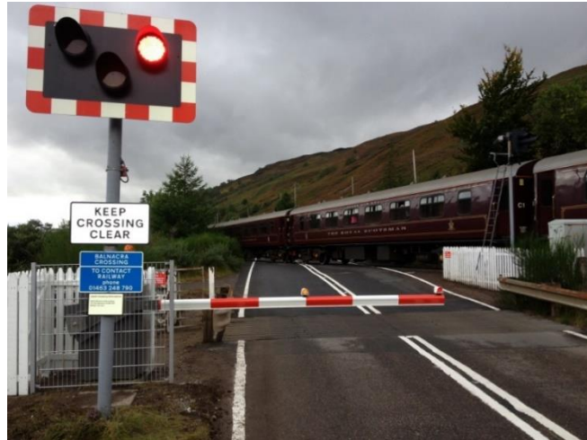
Figure 4-3 An Automatic Half Barrier Crossing
