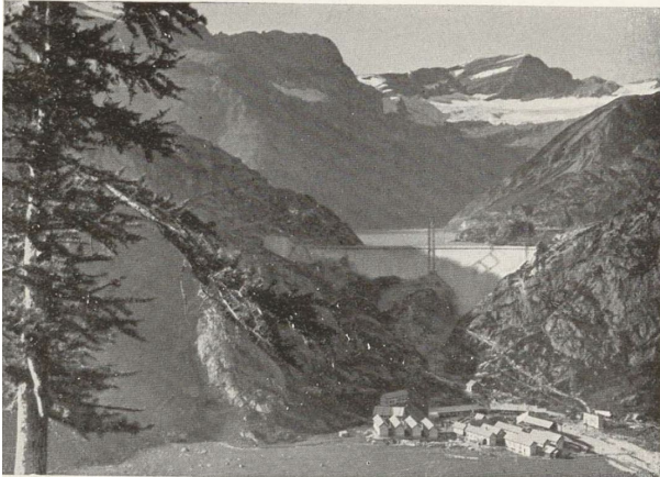
Waterpower plant build in Barberine in 1923 owned by the Swiss Federal Railways with an electricity production of up to 15000kW and an embankment dam capacity of 39000000m 3 .
