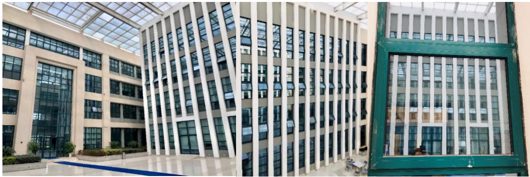
Fig.8. Maintenance Curtain Walls of the Building Atrium in Western and Eastern Facades
