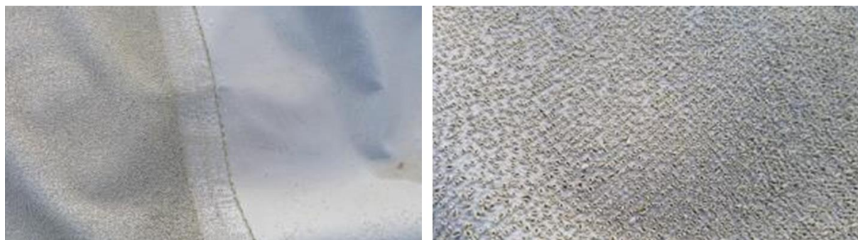
Figure 6: Degradation of a PVC coated polyester fabric due to the exposure to the chemicals of a biogas plant (source: Maco Technology srl).
