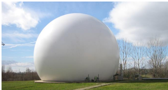
Figure 5: Example of a double-membrane gasholders [6] (source: GTI Covers)
