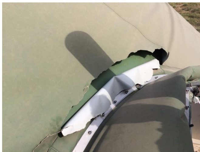
Figure 8: Damage in correspondence of a rigid boundary due to the strong wind and the progressive decrease of the mechanical performance of the coated fabric (source: Maco Technology srl).
