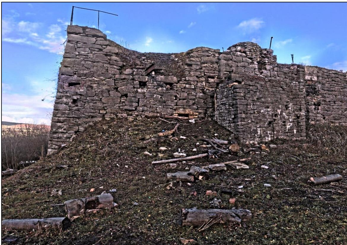
Figure 8-11 Some fallen parts in the SE face.
