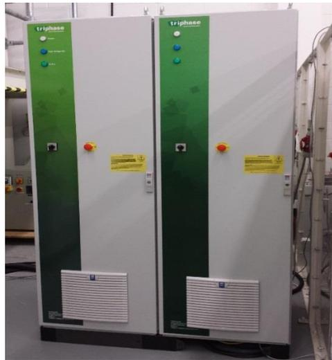
**Fig. 8.3: Triphase Programmable Power/Voltage Supply (Microgrid Source)**
