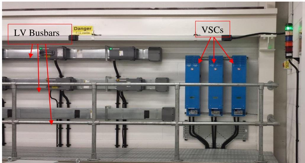
**Fig. 8.2: Three VSCs and the Low Voltage Busbar**
