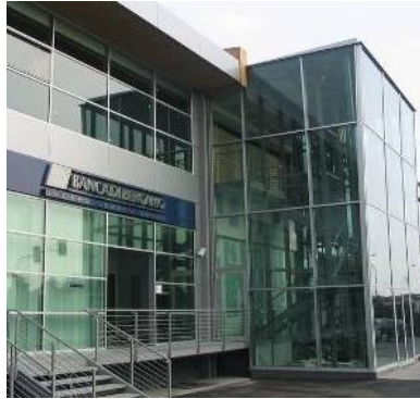
Pressure Plate System (Schuco FW50+)
