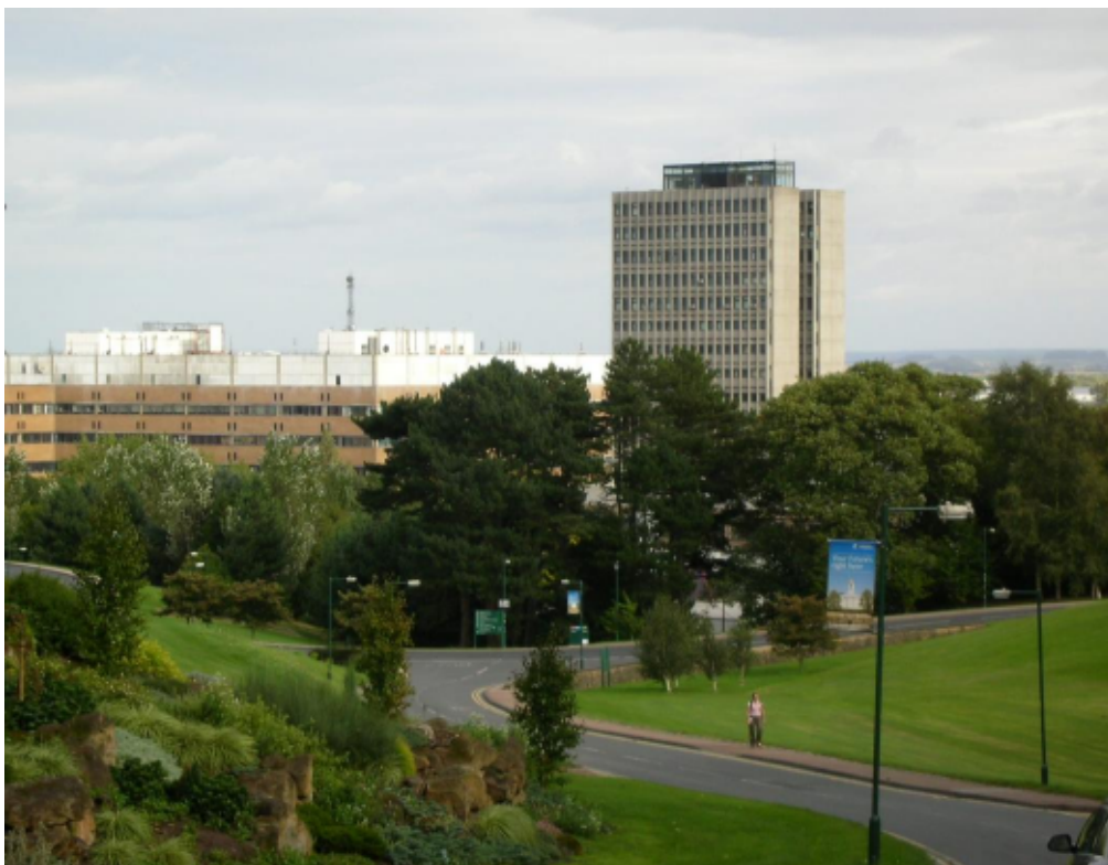
Figure 2.18 View from the west side of the Tower Building
