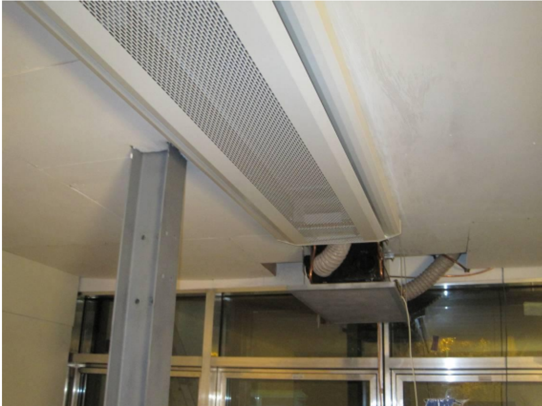
Figure 6.18 View of Heat Exchanger and Active Beam
