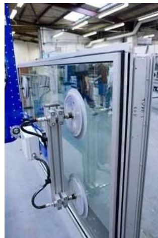
Installation of glazing (notional)
