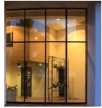
Structural silicon glazed (Schuco FW50+SG)
