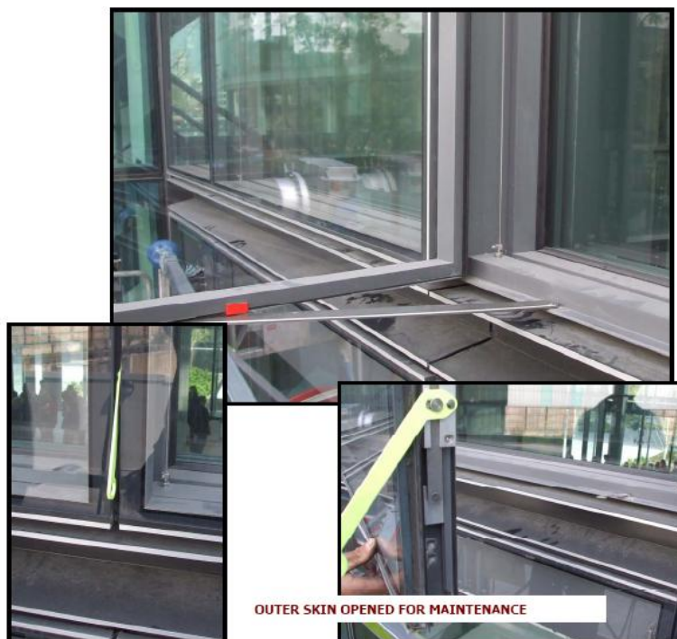
Figure 3.11 Externally access double skin cavity, 7 More London, Foster and Partners, pictures by Lindner Schmidlin (Buro Happold Intranet)
