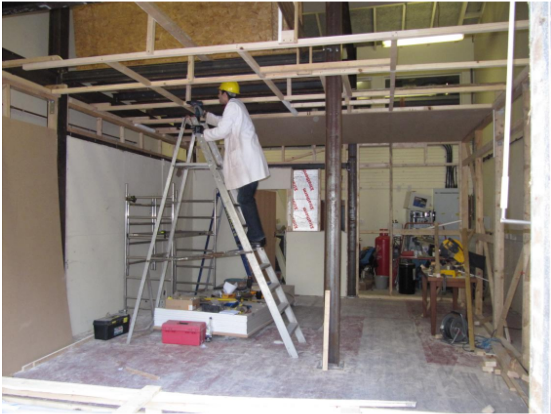
Figure 5.25 Cellular office space being constructed by the author
