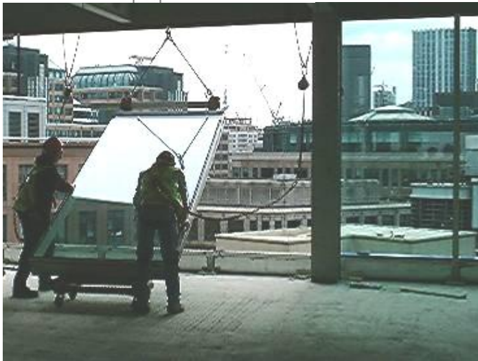
Figure 2.10 Example of a unitised profile (Schueco USC 65 SG) and installation (More Seven, London, Fosters and Partners, 2010)
