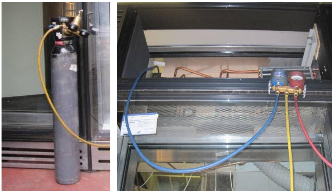
Figure 6.2 Refrigeration charging lines and set-up 237
