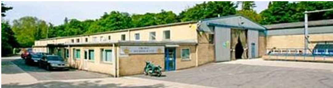
Figure 5.15 External view of works
