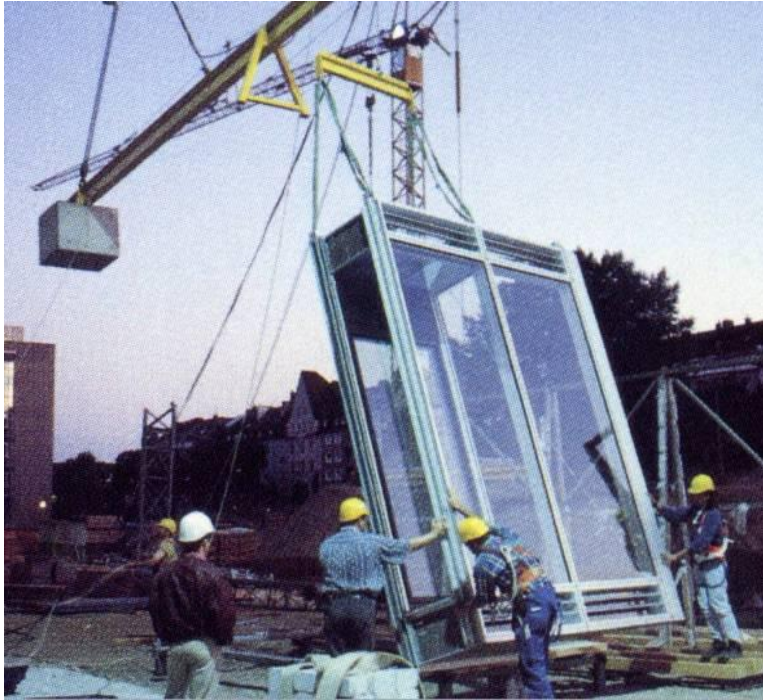
Figure 5.26 External tower crane for facade installation on Stadttor Gate, Dusseldorf, Petzinka, Pink and Partners (photo credit: Josef Gartner)
