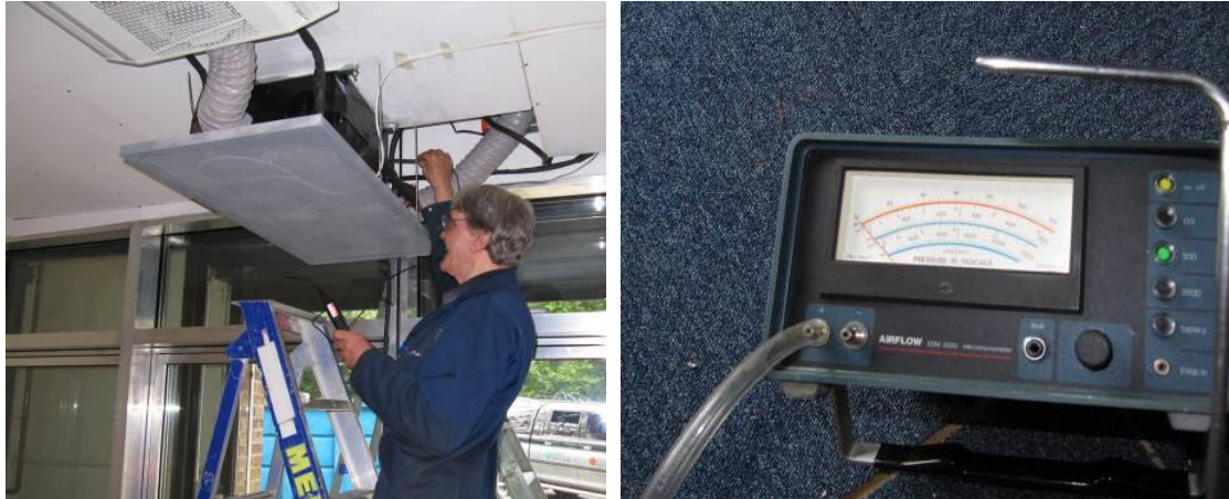
Figure 6.12 Measurement of air velocity and manometer for static pressure
