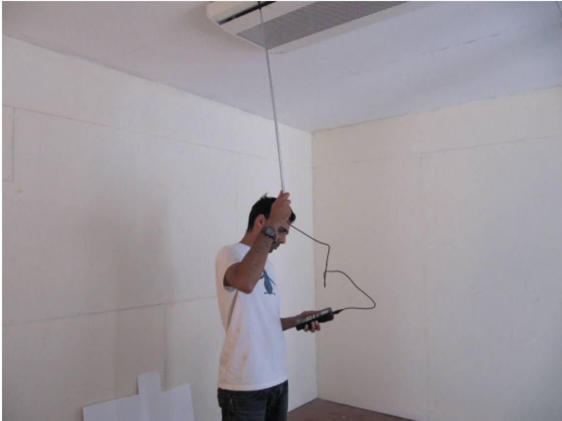
Figure 6.10 Picture of hot-wire anemometer reading being taken for the Active Beam by the author
