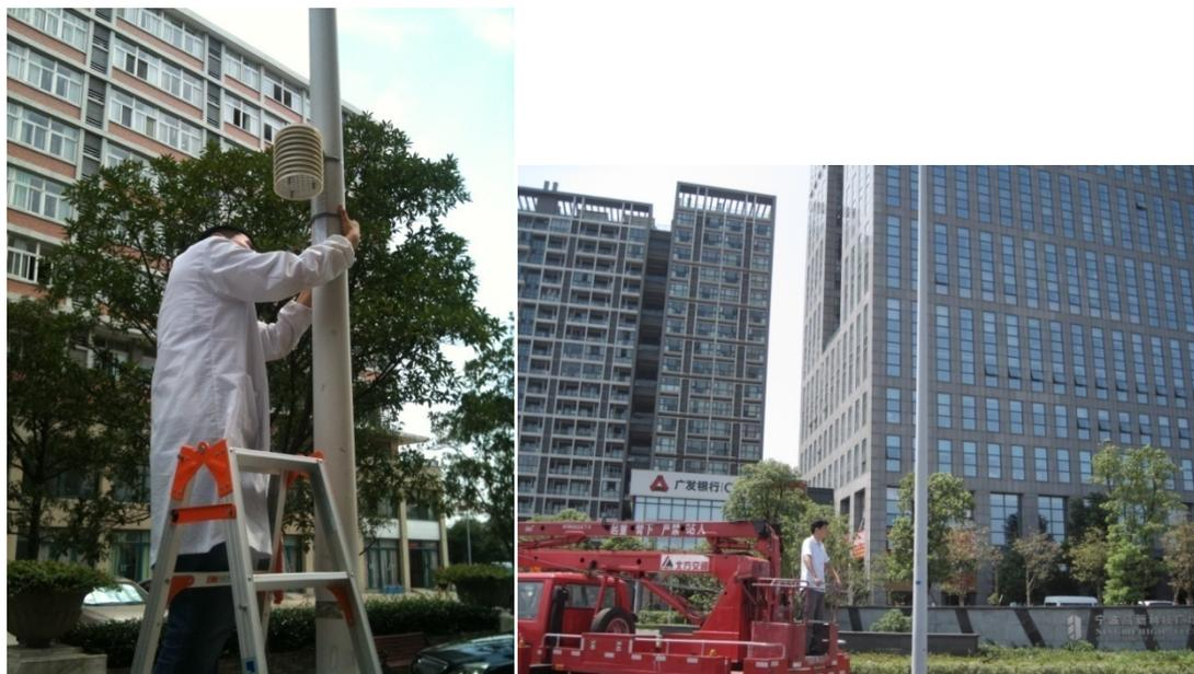
Fig. 4.13: Sensor with radiation shield installation process
