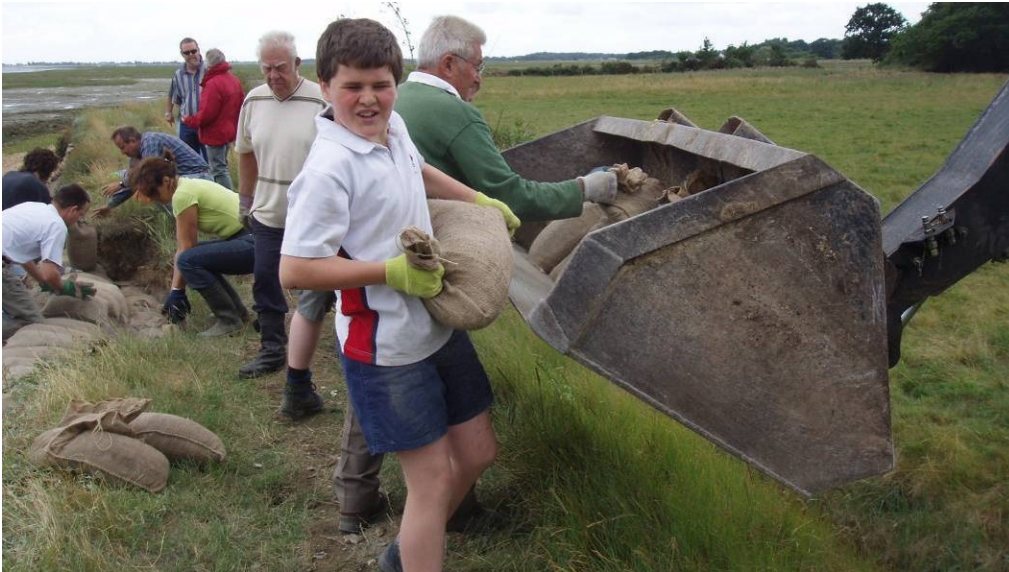
Figure 4-20 Volunteers on crest of sea wall unloading bags from mechanical handler bucket and placing bags (background) 18 July 2009
