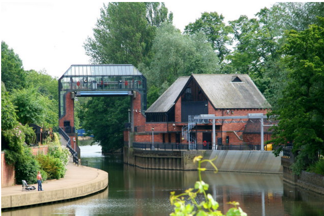
Figure 7-3 The River Foss Barrier as viewed from Castle Mills Bridge, York. (© Copyright David Rogers and licensed for reuse under a Creative Commons Licence. Downloaded 15 th July 2011 from www.geograph.org.uk/photo/866662 )
