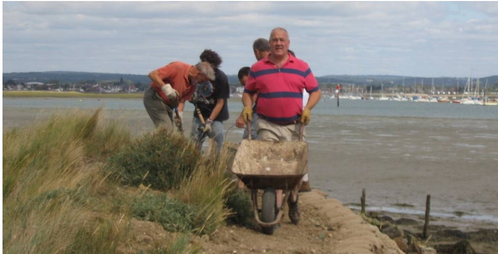
Figure 4-24 Moving and placing clay fill to make up crest of sea wall, 31 August 2009
