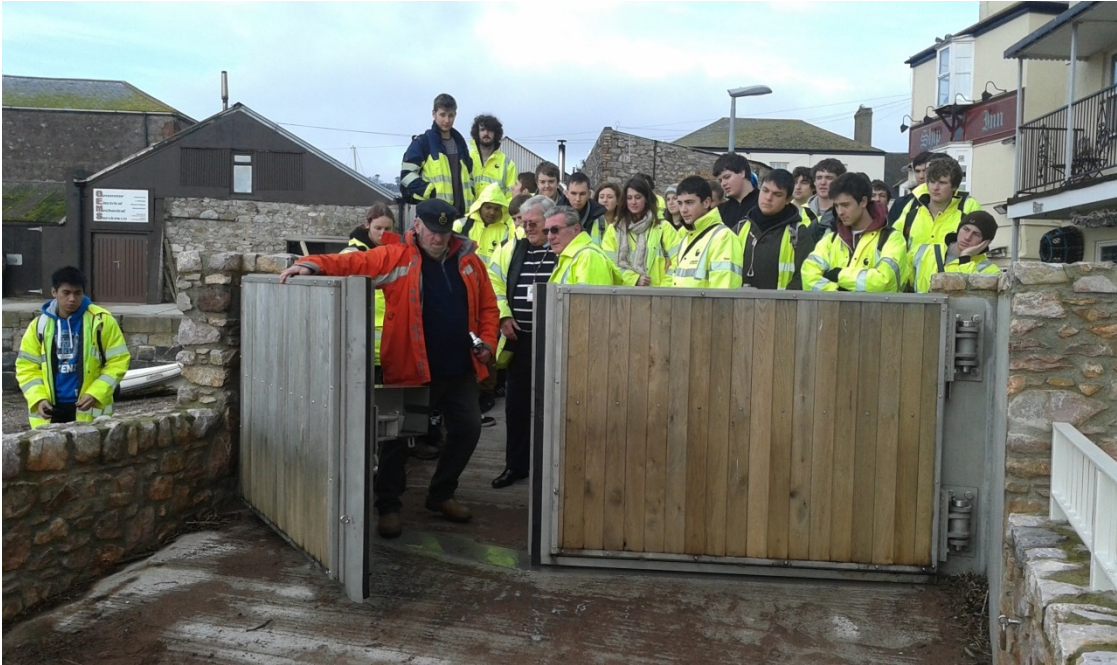
Figure 4-1 Flood gates installed in Teignmouth in 2013
