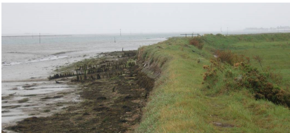
Figure 4-12 Typical view of sea wall (May 2009)
