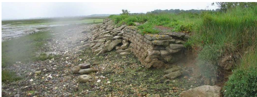
Figure 4-18 Example of existing concrete bagwork walling, including collapsed section in rearground and eroded bank in foreground
