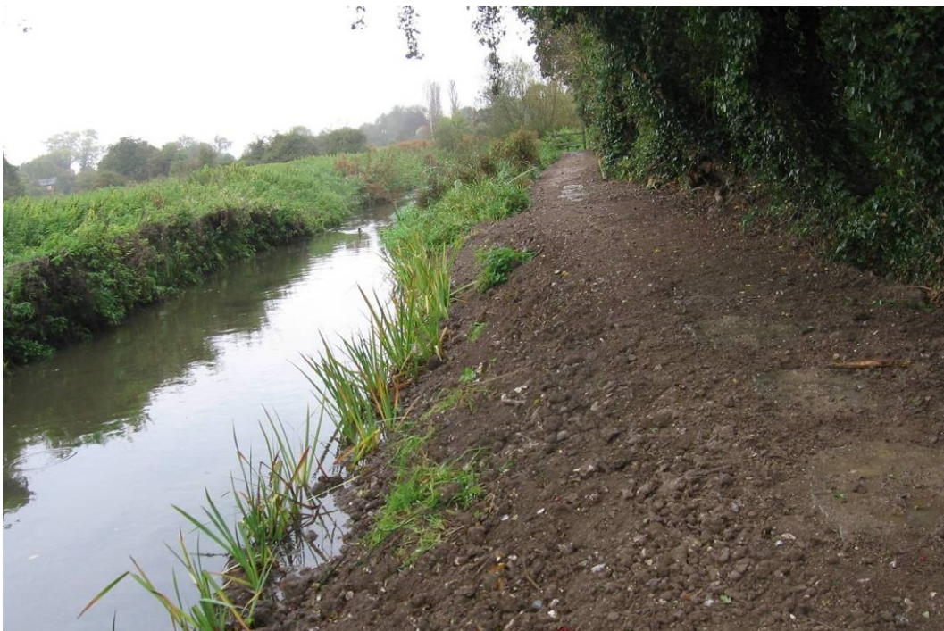
Figure 4-6 (a) Installing coir rolls at base of bank to provide stabilised toe to (b) new bank slope and encourage water line vegetation, September 2008 (Courtesy Hanneys Flood Group)
