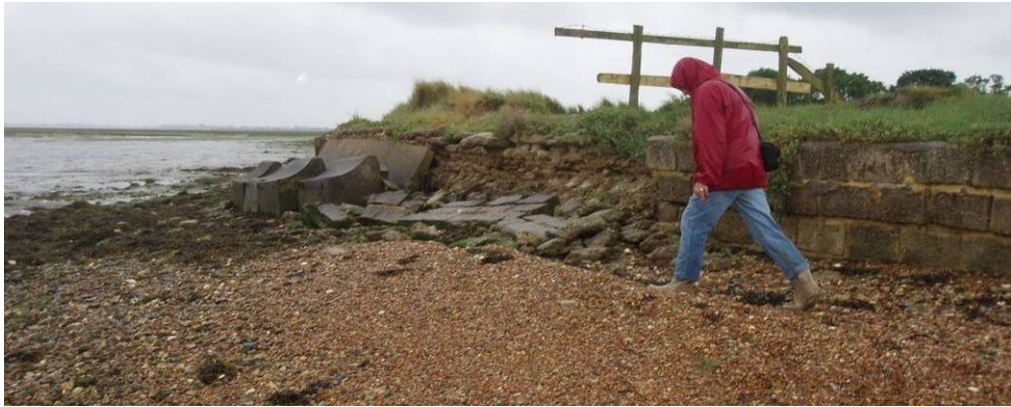
Figure 4-15 Example of collapsed concrete blockwork wall facing.
