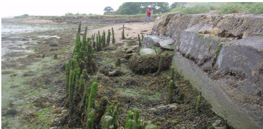
Figure 4-14 Example of mass concrete wall with timber stakes exposed by eroded beach
