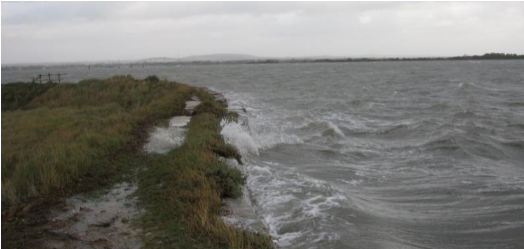
Figure 4-29 Sea conditions at Northney seawall 14 th November 2009 (Courtesy Judy Clark) Notes on conditions: Pressure 998mb; high tide nominal height +4.7m CD/ +2.0m OD, actual maximum water level about + 2.5 to 2.6m OD. i.e. at least 0.5m storm surge.
