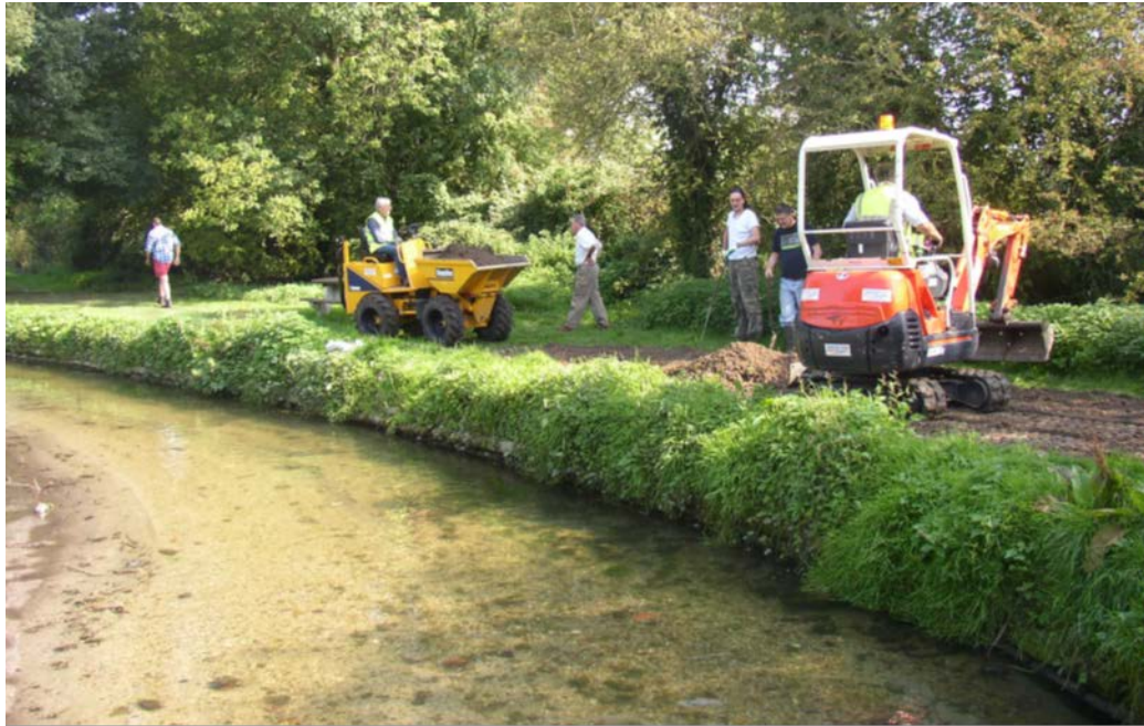
Figure 4-5 Letcombe Brook, showing commencement of low bund construction by Hanneys Flood Group, September 2008 (Note drop in water level compared with previous figure following weed clearance) (Courtesy EA)
