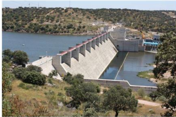
(a) Downstream view from the right side
