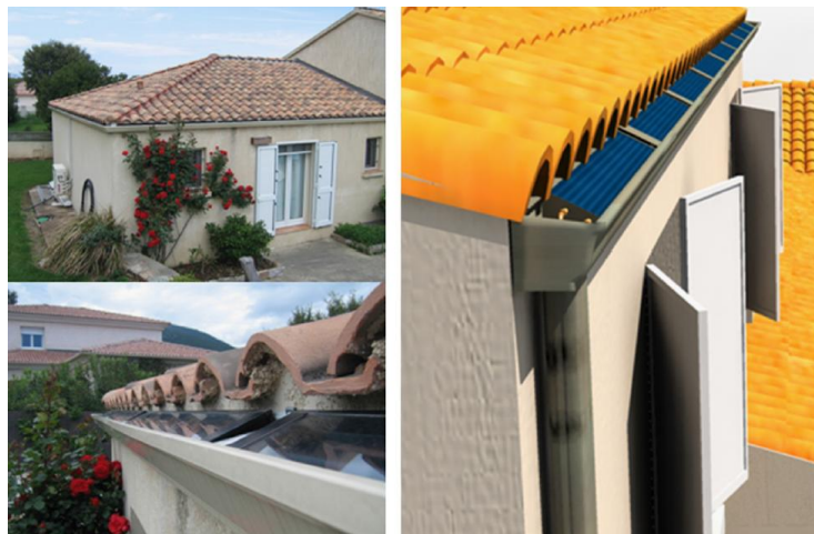
Figure 2.2.18 The view of a transpired solar collector (Notton et al., 2014)
