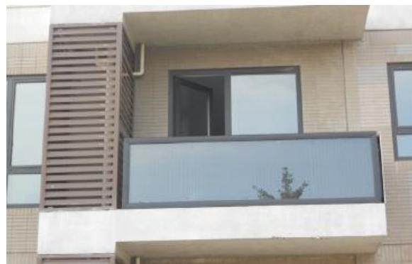
Figure 2.3.11 Solar ceramic collectors as balcony railings (Yang et al., 2013)
