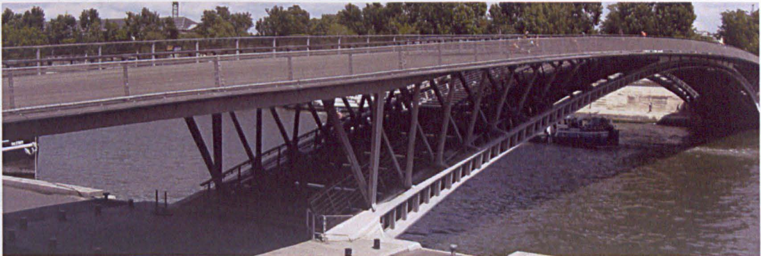
Figure 2.1: Pont de Solférino, Paris (image after [1]).
