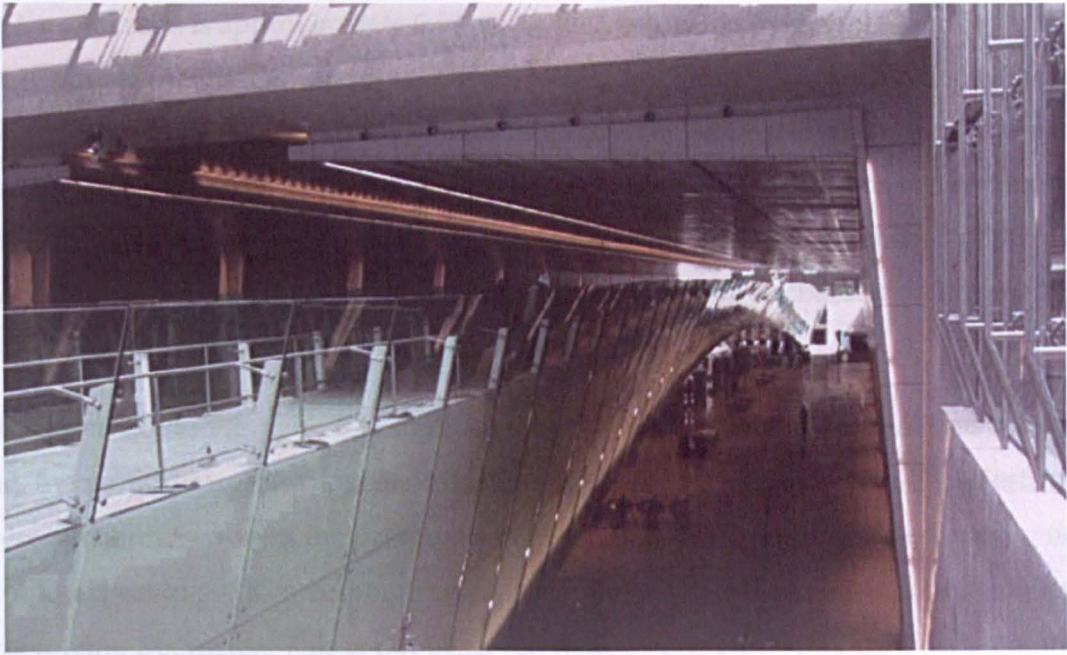
Figure 2.9: Changi Mezzanine Bridge (CMB), Singapore [6].
