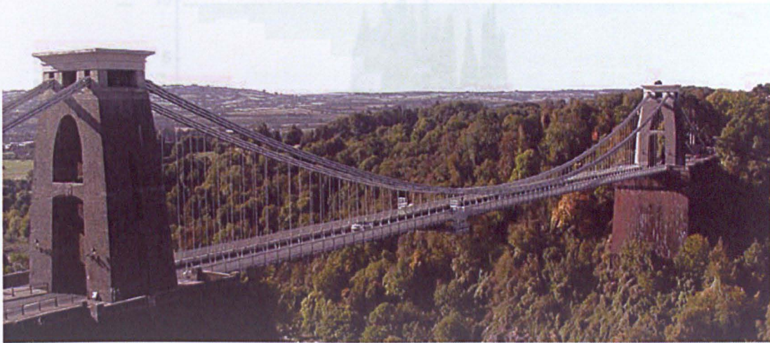
Figure 2.14: Clifton Suspension Bridge, Bristol (image after [1]).
