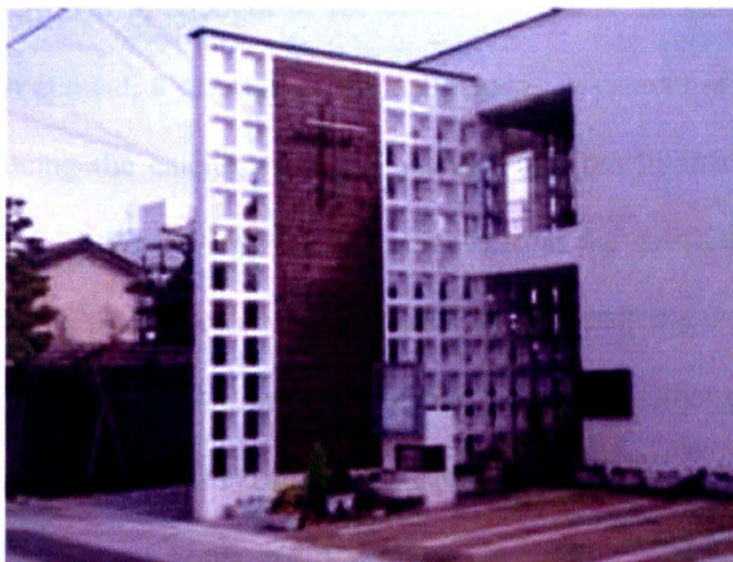
Figure 2.1 This lattice wall was cast with SCC from only one point at each floor Source: Okamura and Ouchi, 2003a
