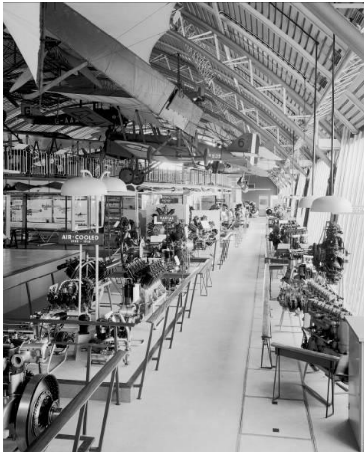
Figure 132 A 1960s photograph of the Aeronautics Gallery on its opening in July 1963. Like the Sailing Ships Gallery on the floor below, O'Dea's display ideas were innovative and ambitious. Here the planes hover above the floor, hanging from the hangar-like ceiling alongside the raised walkway for visitors. (© Science Museum / SSPL).
