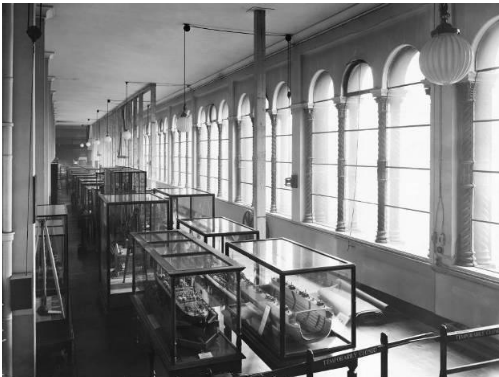
Figure 53 A photograph of the closed Gallery 13 (ship collections) in the South Galleries 1862 buildings in November 1932 before they were moved into the new East Block. Notice the wooden support beams holding the roof (© Science Museum / SSPL).
