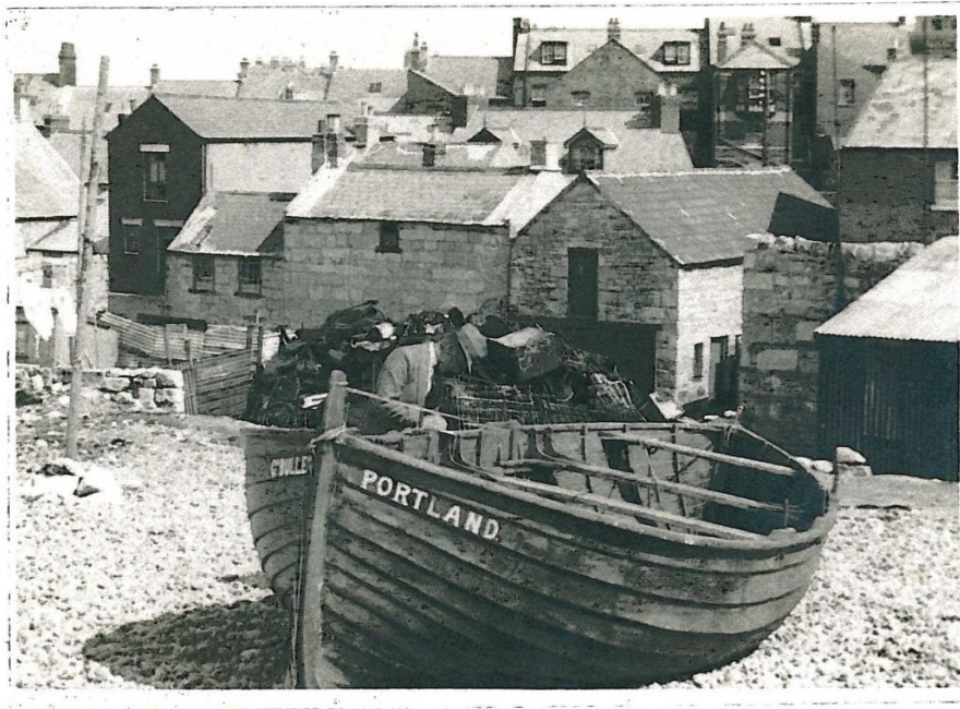
Figure 67 An image of photographs of an individual (possibly Major Castle Smith) taking lines of a rotting Portland Lerrit on Chesil Beach. He used these lines to make the model. (SMD SMD T/1938-461).
