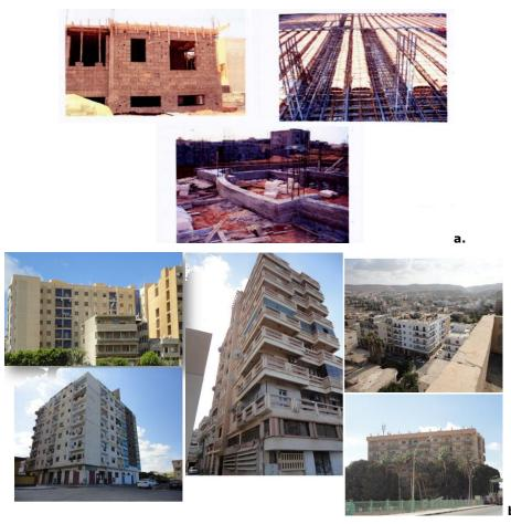
Figure 5.7: a) Building materials and construction system used in Libya in general including the case study Danah. Concrete floors & roofs, steel and hollow concrete blocks \_ b) Photos shown examples of city mid-rise buildings (B1, B3, B6, B8 & B10) as well as shown finishing materials \_ source: Site visits photographs, summer 2010
