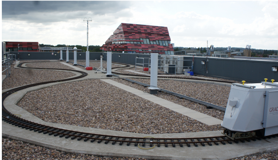
Figure F.1 – A view of the NGB Roof
