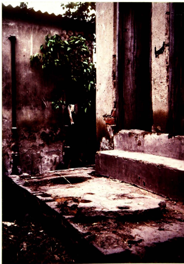
CMDA constructed septic tank latrines with crumbling mortar and missing manhole covers
