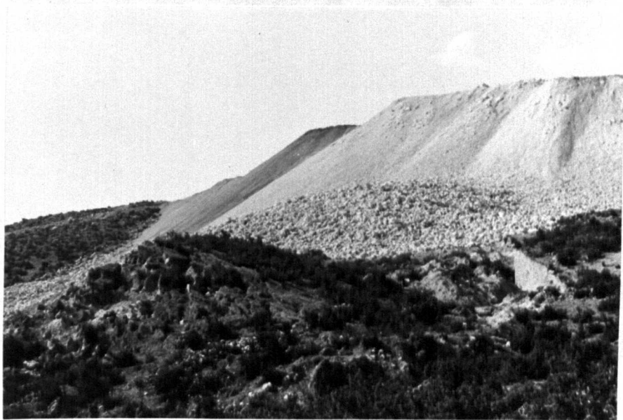
Plate 112. Land-slides caused by the weight of the waste dumps near the Hisarcik opencast mine.
