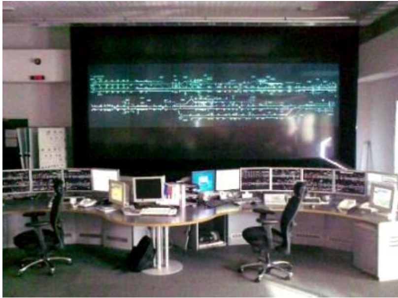
FIGURE 7-3: MANCHESTER SOUTH SIGNALLING CONTROL CENTRE
