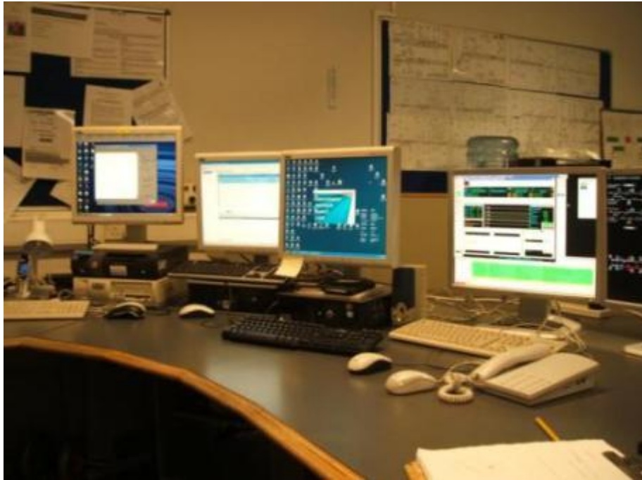
FIGURE 2-4: MANCHESTER SOUTH MAINTENANCE CONTROL CENTRE
