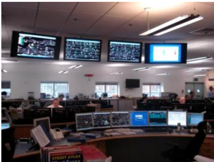
FIGURE 7-8: LONDON NORTH EAST NATIONAL CONTROL CENTRE
