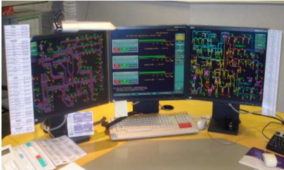
FIGURE 2-6: ELECTRICAL CONTROL ROOM SCADA
