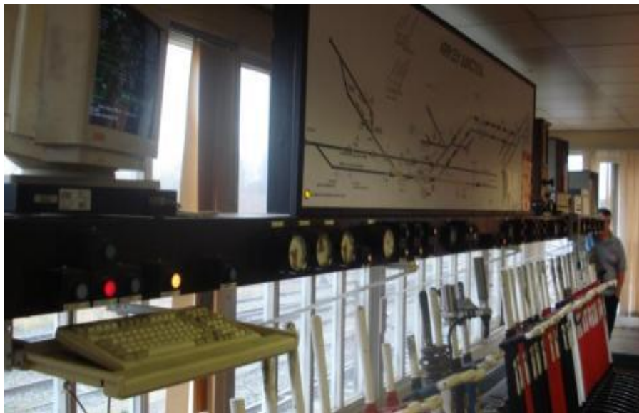
FIGURE 2-1: LEVER FRAME SIGNAL BOX
