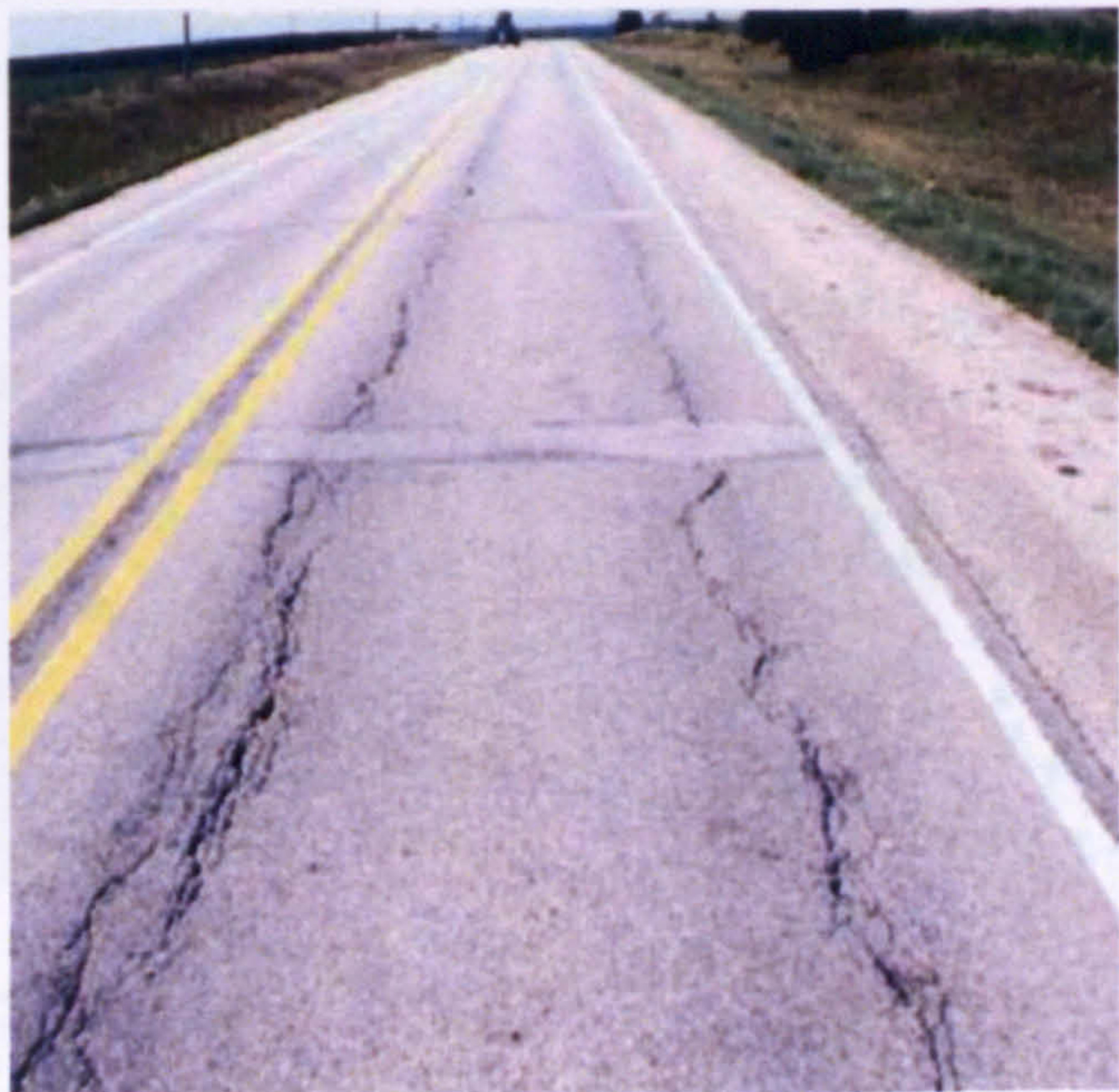
Figure 2.8. Fatigue cracking in wheel paths
