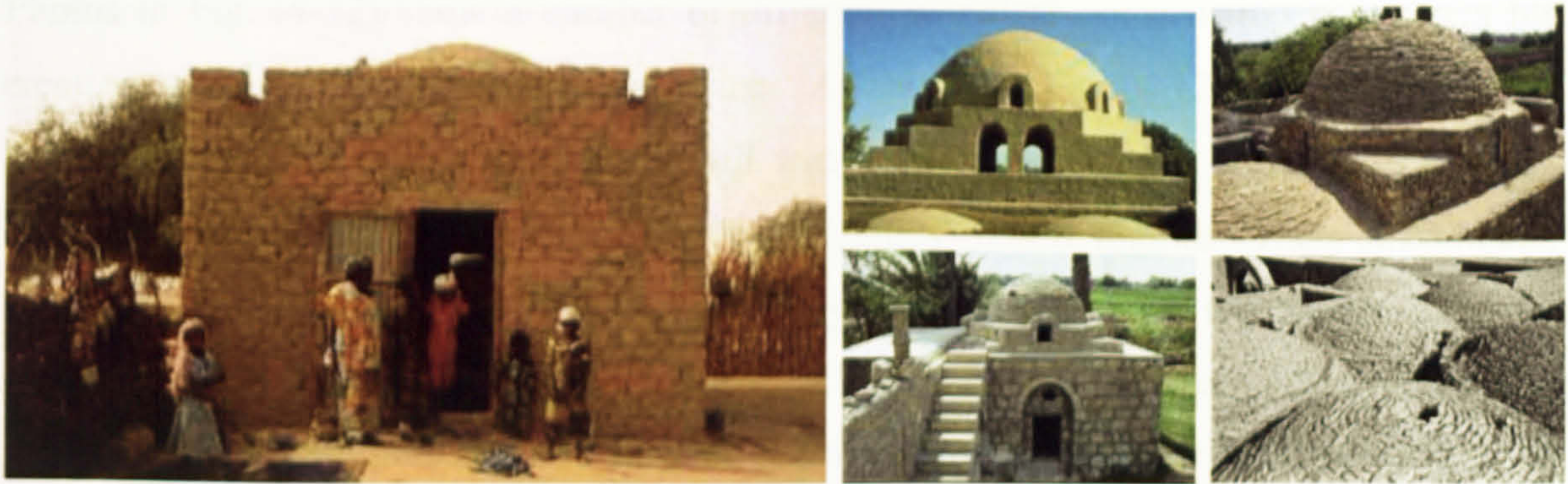
Figure 4-10 Different Woodless and Mud-Bricks Domes Covering Different Plans
