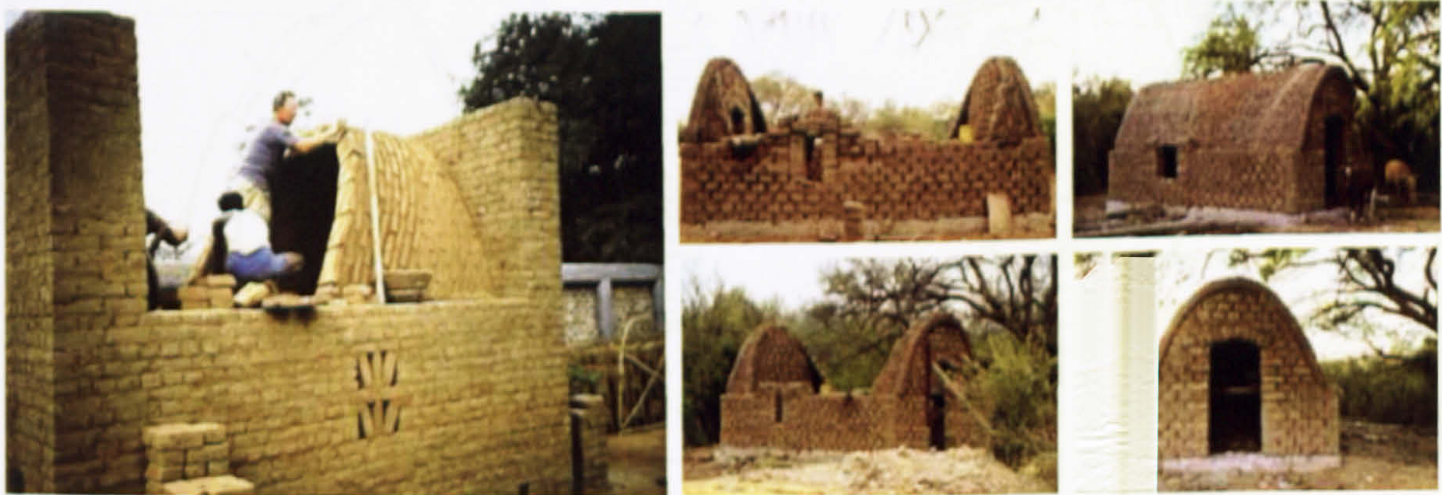
Figure 4-5 The Nubian Way for Erecting Vaults, Source: www.canelproject.com [14]
