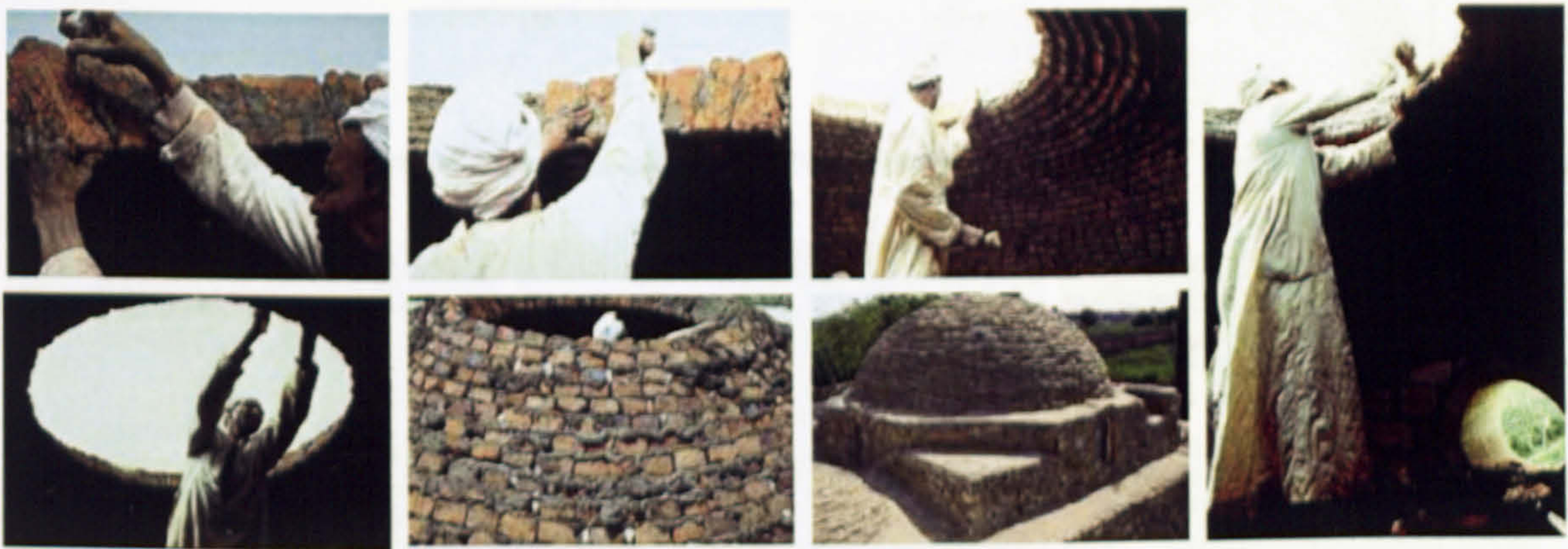
Figure 4-7 The traditional Process of Erecting Woodless Mud Bricks' Domes Source: ArchNet Digital Library [13]
