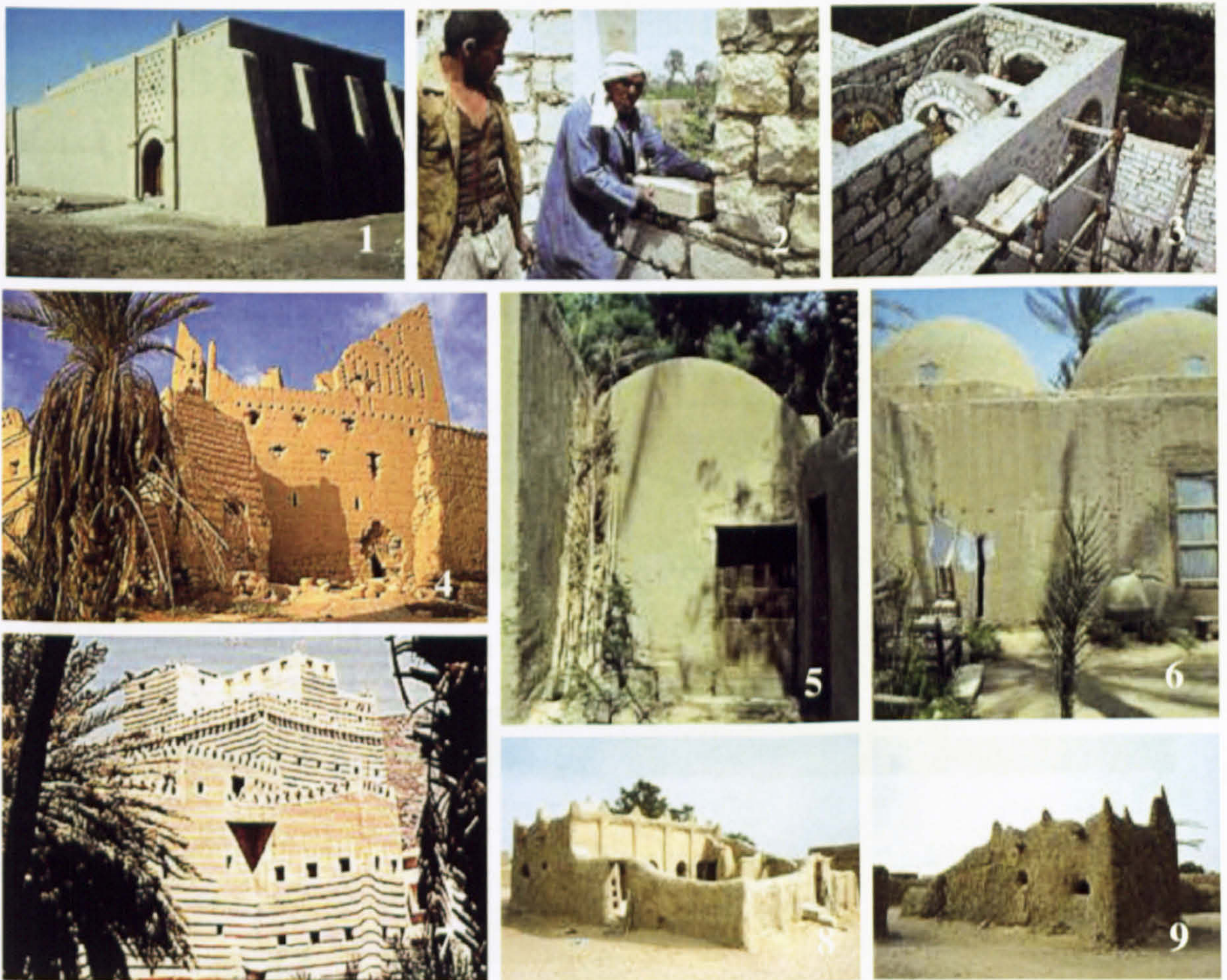
Figure 3-8 Photos Depicting Thick and Massive Walls with Different Construction Materials, Source: ArchNet Digital Library [9]
