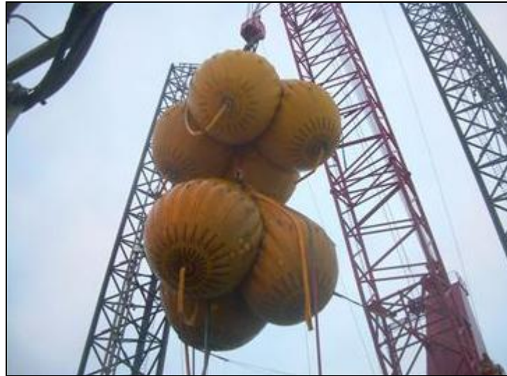
Fig. 2.18 Seven 35t water load test weights configured in one set of four and one set of three [81]
