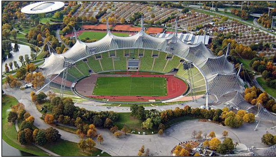
Fig. 1.7 The membrane roof on the Olympiastadion in Munich [39]
