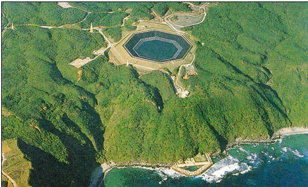
Fig. 2.5 Pumped hydroelectric energy storage plant using seawater [57]
