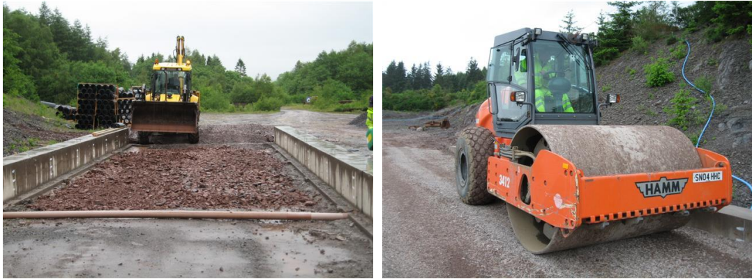
Figure 4.15 – (a) Levelling of the floor (b) Compaction works at the top of the base layer
