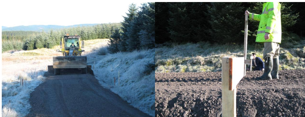
Figure 4.12 – (a) Reference section construction at Castle O'er. (b) Layer thickness monitoring during construction
