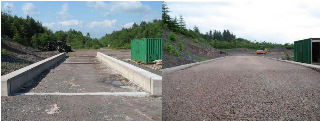
Figure 4.16 – Ringour Testing Facility – view of the test section before and after construction of the test pavement
