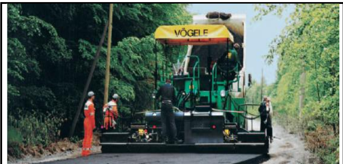
Figure 2.7: Cold Recycled Mix Placement (Wirtgen, 2005)
