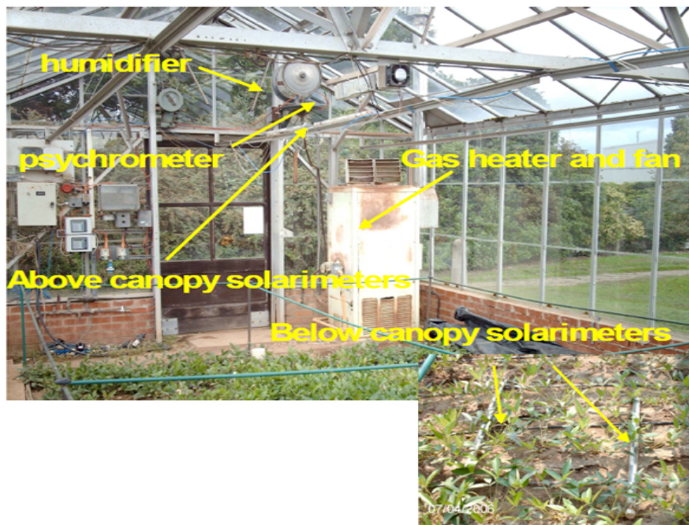
Plate 3.2 Glasshouse facilities and structures used to control the inside environment.
