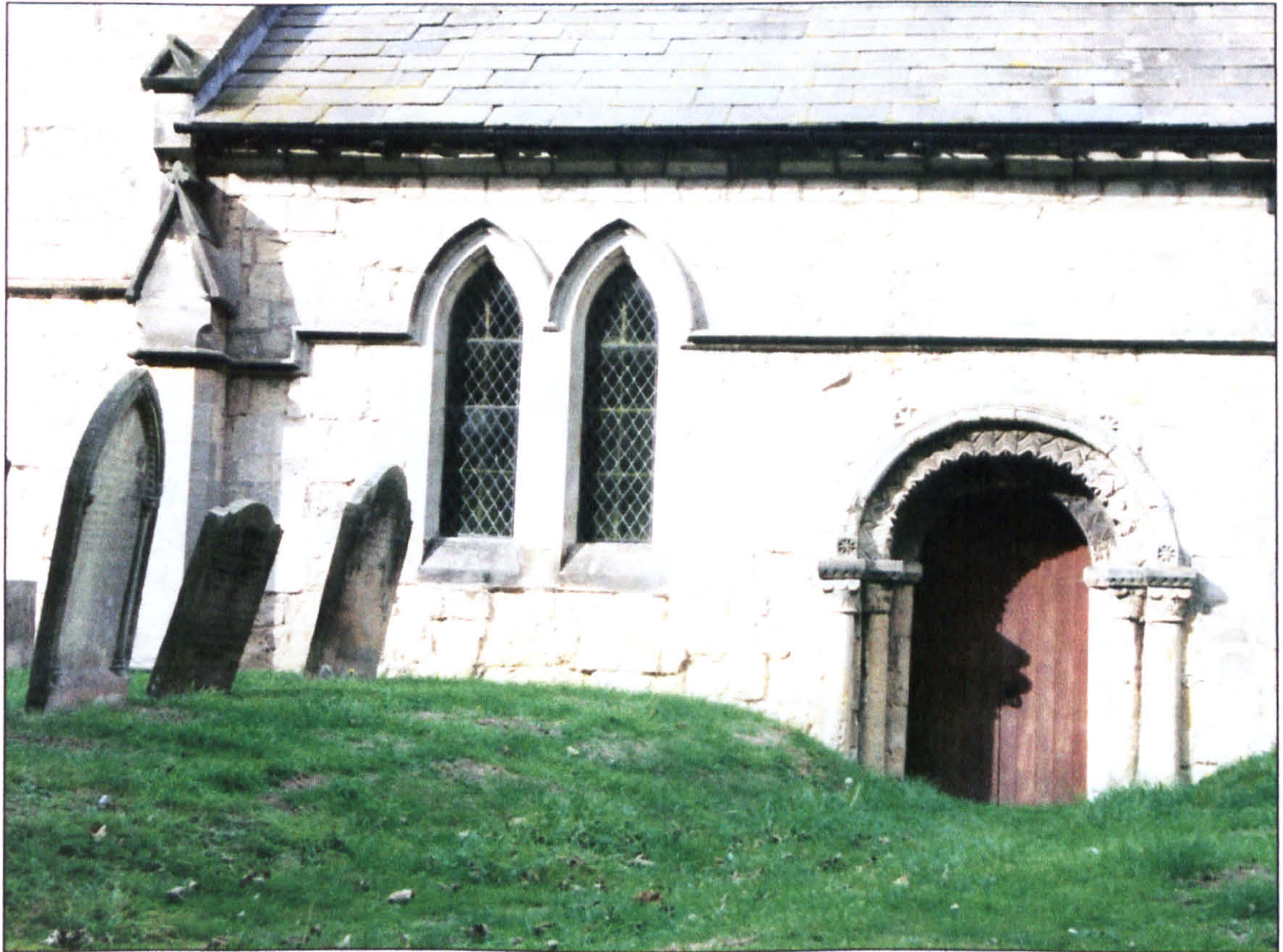
Figure 4.11 Norman masonry and doorway of three orders at North Dalton.
