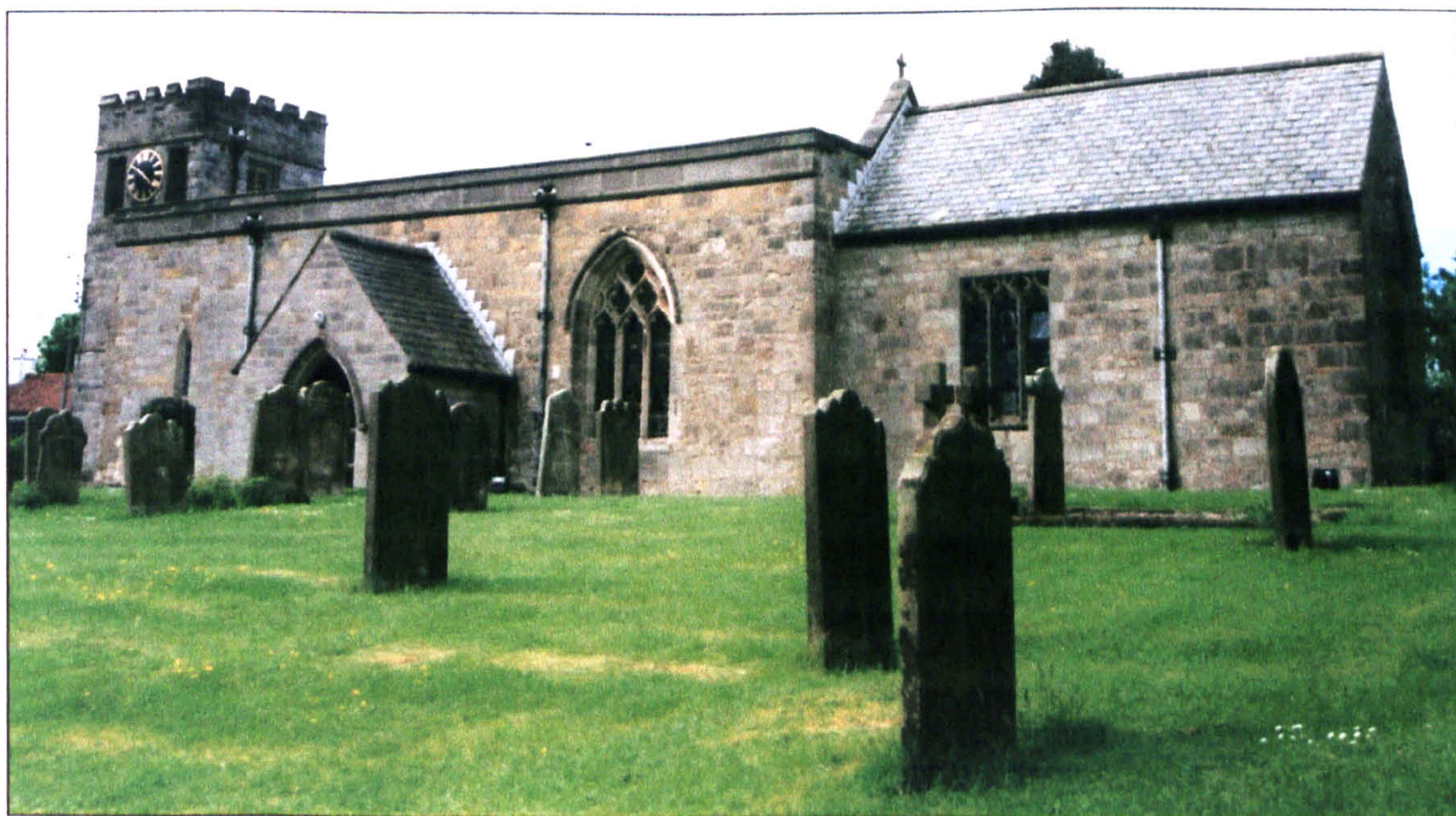
Figure 6.22 Reticulated tracery in the south nave wall, Thwing.
