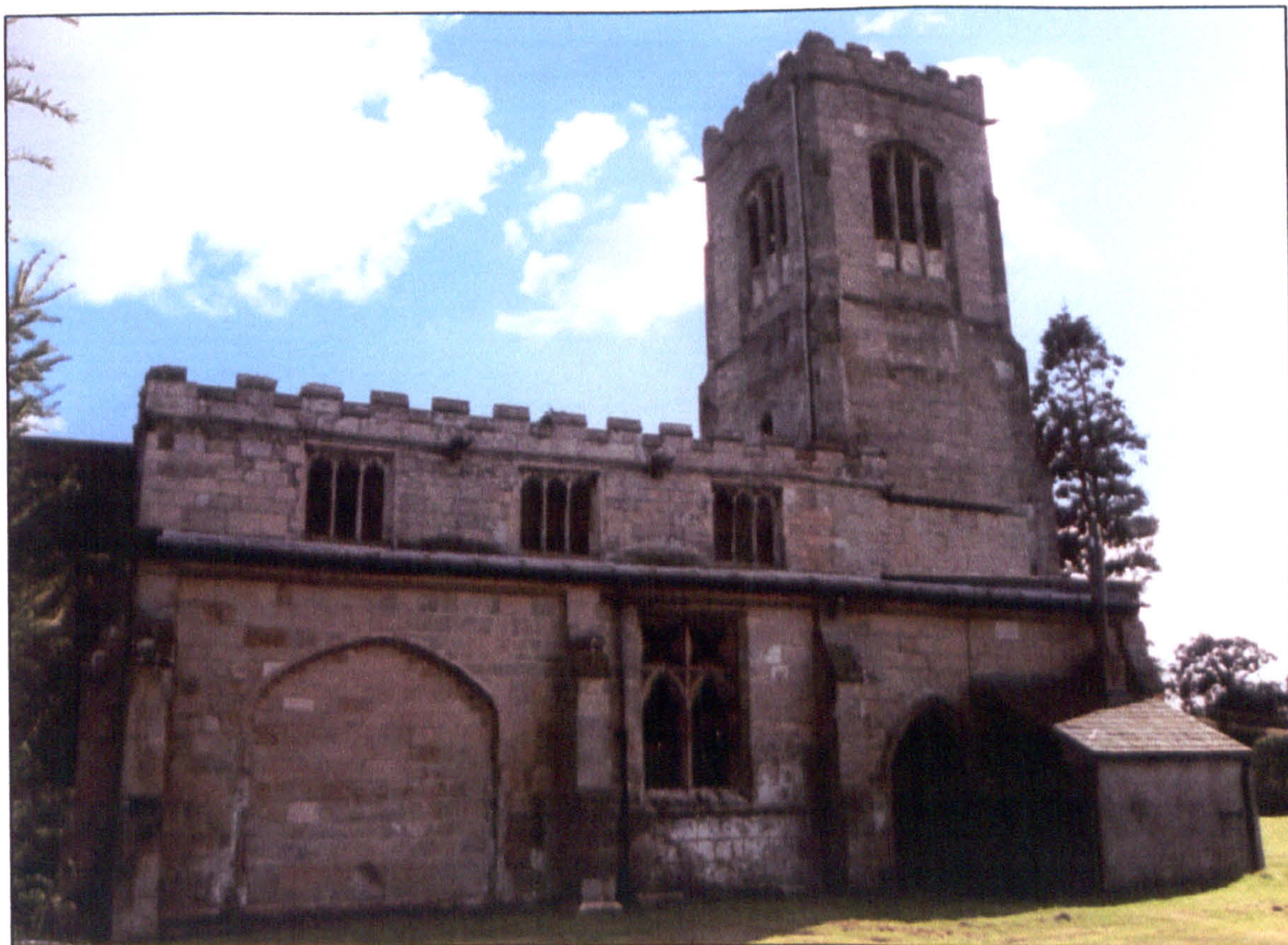
Figure 6.24 St Martin, Burton Agnes from the north, showing Tudor arch to demolished north chapel, clerestory and embattled parapet on the nave.
