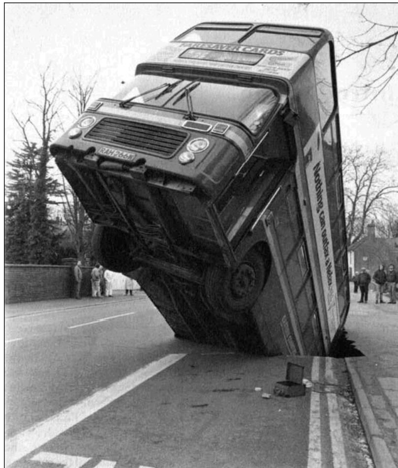
Figure 1.1: An example of sudden collapse resulting from unknown underground voids (Waltham, 1989).
